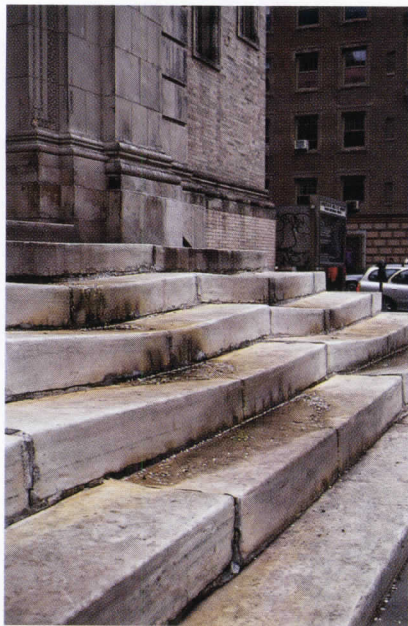
No skateboarders will attempt these stairs, which suffered the effects of weathering and an inadequate substrate. The treads were also not properly angled to prevent ponding.
