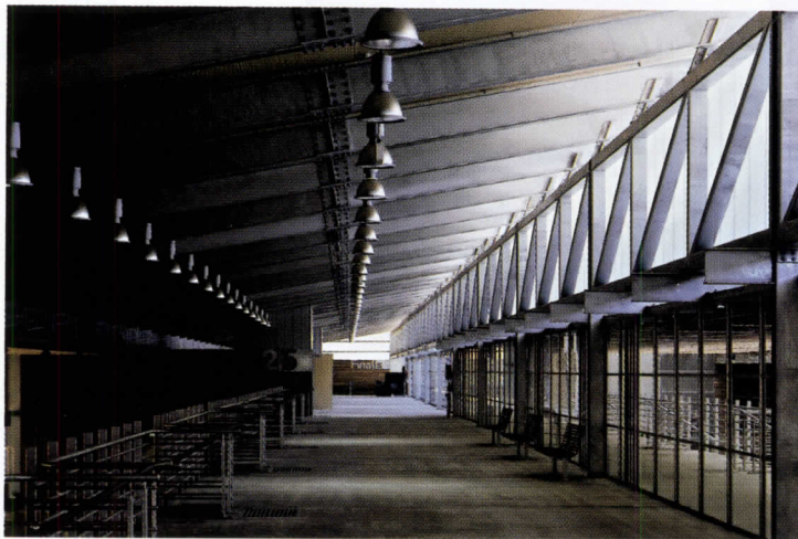
Sydney's new $30 million Shooting Centre, by Gazzard Sheldon Architects, will incorporate shooting ranges as well as covered spectator facilities.
