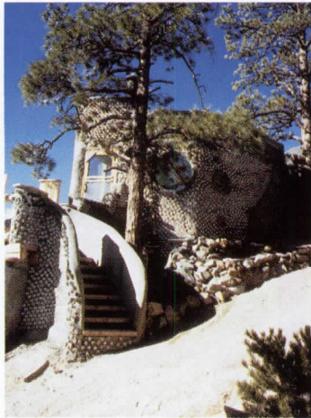
Examples of Reynold's Earthship houses, constructed from beer cans, bottles, and tires molded into adobe.
