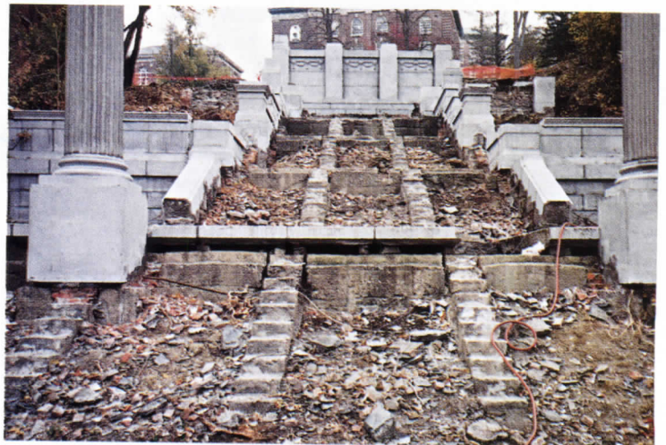
In Troy, N.Y., a 93-year-old stairway leading from the town center to RPI was restored (top) by Architecture Plus after years of neglect (bottom).
