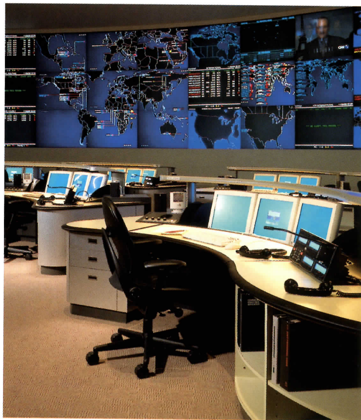
HOK designed the consoles to function like automobiles. Each has its own HVAC system and audio system. The work-surface height is adjustable.
