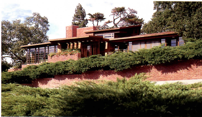
Massive unreinforced chimneys, long window walls, and an open plan (above and left) made the repair and seismic upgrade of the Hanna House difficult.
