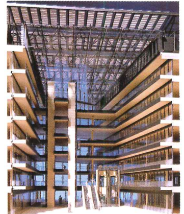
Courtyard roof of photovoltaic cells
