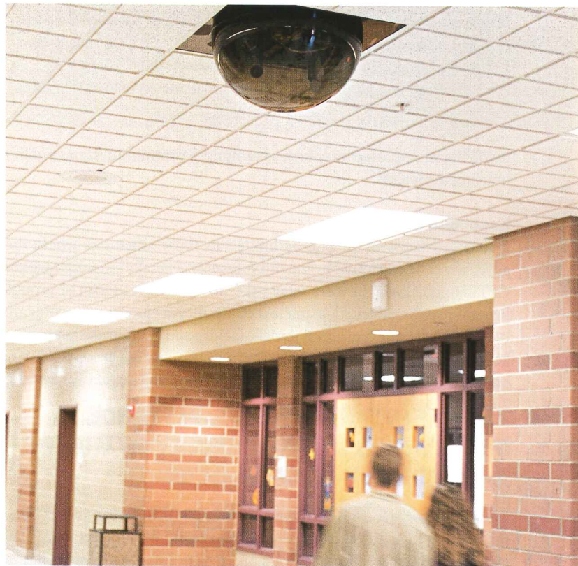
Security cameras monitor activity in hallways and all public areas of Chesterton High School and feed images to a central security office.
