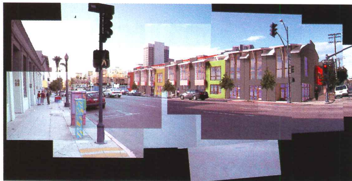
"ROWhomes on F" by deFreitas deSign are 17 structurally independent units.
