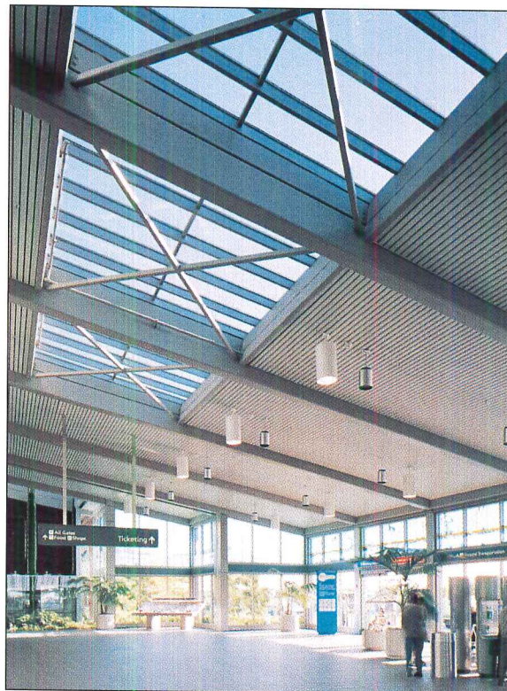
Photo: Sacramento International Airport, Terminal A Architect: Dreyfuss & Blackford Architects Photo: Cathy Kelly Architectural Photography A/D FIREFILM® II on structural steel.
