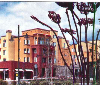
Project: Bridgecourt Location: Emeryville, Calif. Architect: McLarand, Vasquez & Partners Client: Catellus Residential Group
