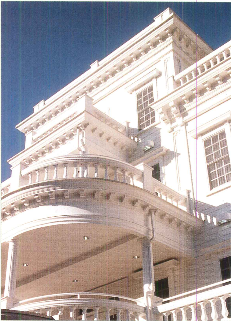
Incorporating dozens of urethane balustrade systems, corbels and brackets from Style Solutions, the Riverview Health Care Center resembles a stately hotel.
