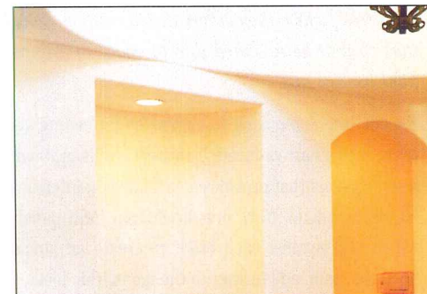
Flexible 1/4-inch-thick SHEETROCK Brand Gypsum Panels facilitate curved drywall applications.
