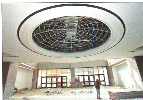
The USG Drywall Suspension System saved hundreds of man-hours and ensured perfect results on the construction of 19 domes in Regent Auditorium, Pensacola.
