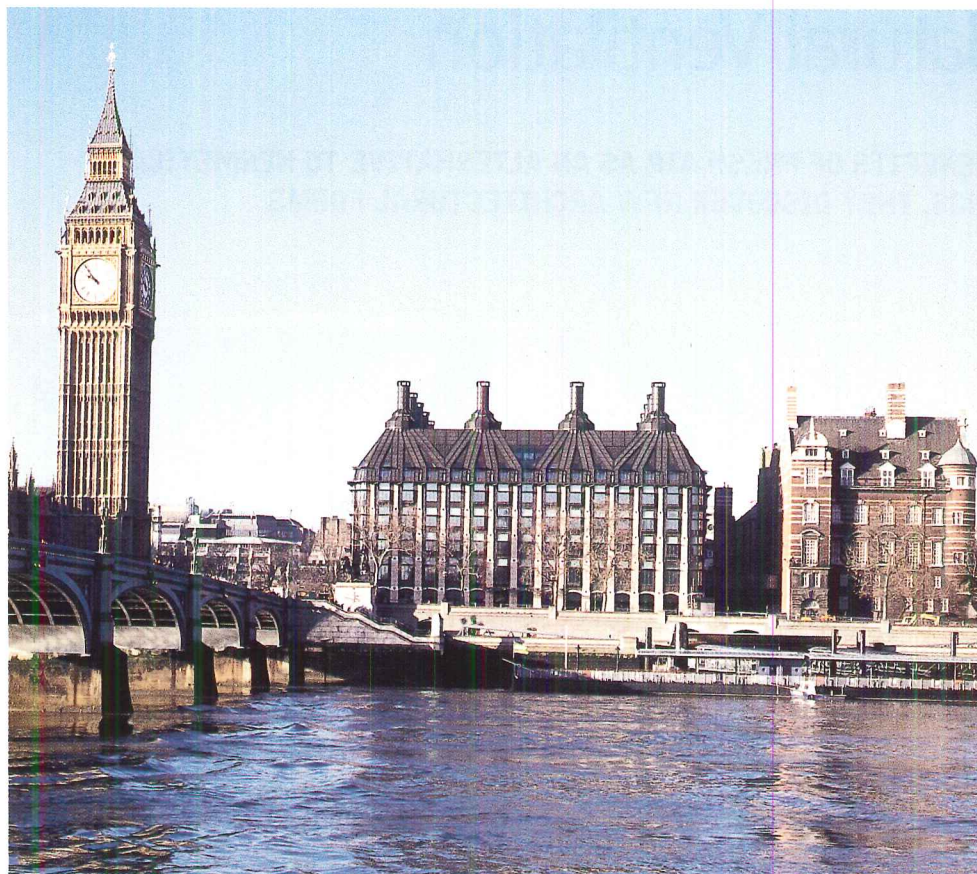
Portcullis House (left), across from Big Ben, houses offices for members of Parliament. The wall cavities and ducts, articulated on the facade, actually diagram the path from the main block to the rooftop. Fresh air is delivered to the offices (above) via a plenum under the floor. Solar radiation is absorbed by dark blinds located in the ventilated cavity of the triple-glazed bay windows.
