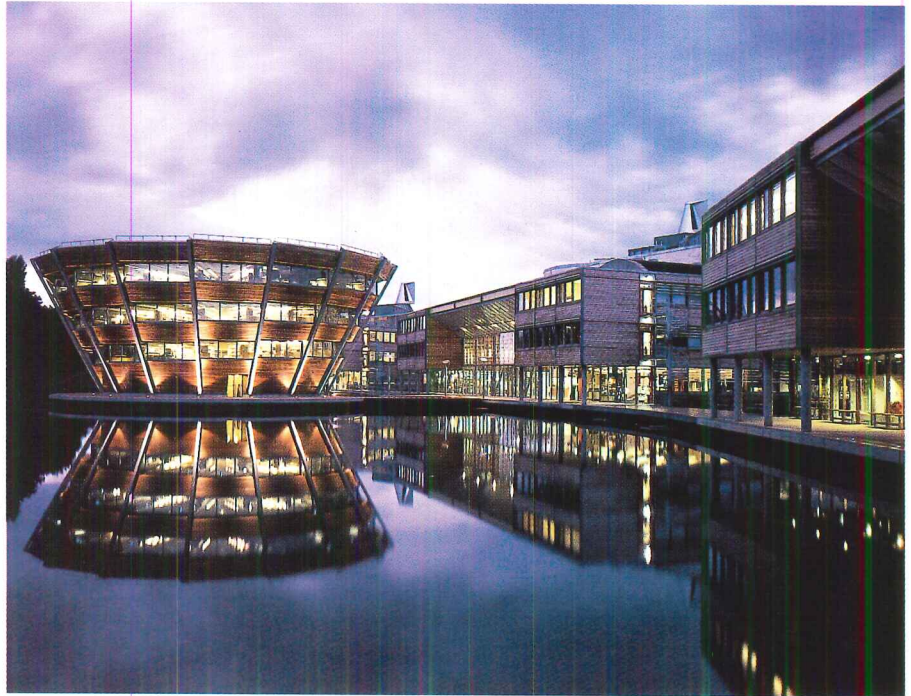
Tower-top cowlings, which can be seen above the buildings, help draw fresh air through the offices at the Jubilee Campus at Nottingham University in the U.K.
