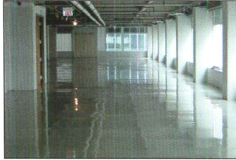
Approximately 525,000 sq. ft. of gypsum concrete underlayment (shown freshly poured) was applied over the existing floors throughout the building.
