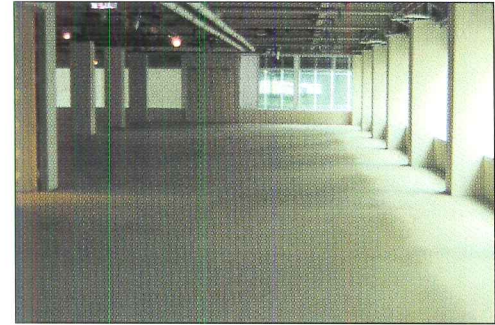
The new gypsum concrete underlayment provides a smooth, even surface, ready for floor finish material installation. The entire application was completed for less than half the cost of using a portland cement-based product.
