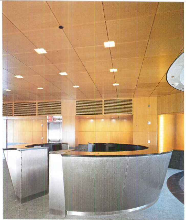
A custom beech perforated-wood ceiling was used in conjunction with non-woven acoustical fabric for this office space in Los Angeles.
