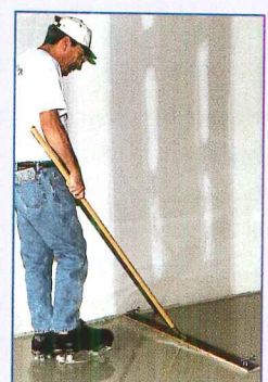
The underlayment was screeded to the thickness of the elevation pins to achieve a smooth, even surface.
