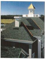
Utilizes CertainTeed's exclusive Super Shangle® construction with two full-size base shingles, resulting in virtually four layers of shingle protection and 8-inch exposure when applied. This super-heavy-weight fiber glass shingle (355 lb. per square) also features a unique chamfered cut for scalloped appearance. UL Class A; lifetime limited, transferable warranty; algaeresistant UL Certified to meet ASTM D 3462.
