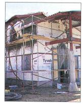
Dupont Tyvek® Commercial-Wrap® is engineered to stand up to the rigors and demands of commercial construction. Tyvek also helps reduce moisture within walls, therefore is one of the ways to help reduce mold and mildew. The properties of Tyvek® do not allow mold and mildew to grow on it. Tyvek® CommercialWrap® can even take up to 9 months of UV exposure and we also have a product specifically engineered for your stucco needs.
