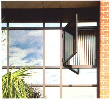
Fixed and movable features such as vertical blinds shown above can block and reflect direct sunlight entering through windows.
