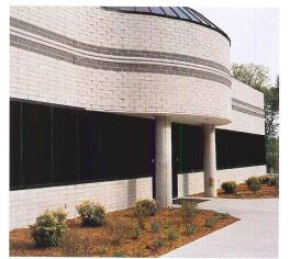
Coca-Cola Bottling Company of Northern New England, Inc., Londerry, NH Architect of Record/Engineer: Stahlman Engineering Corporation, New London, NH Accent Panels: 3 <sup>5</sup>/<sub>8</sub>" x 23 <sup>5</sup>/<sub>8</sub>" x 3 <sup>5</sup>/<sub>8</sub>", #M115, #M1428 Finish: Tudor®
