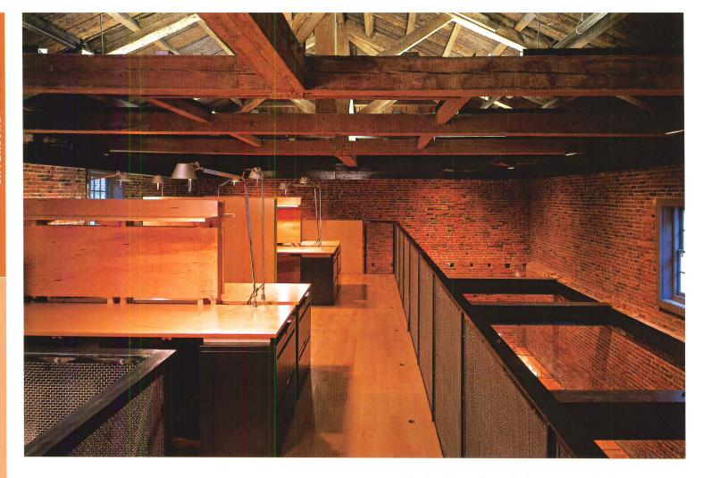
The mezzanine (above) adds nearly 500 square feet of floor space. Steel beams shore up the brick walls, which were 5
