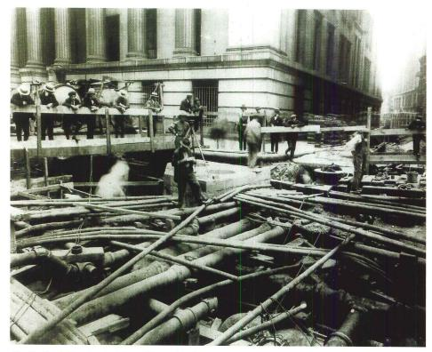
Peeling back the street surface of Lower Manhattan in 1913 revealed a tangled web of pipes and ducts, much of which is still part of New York City's complex infrastructure, and has been for over 100 years.
