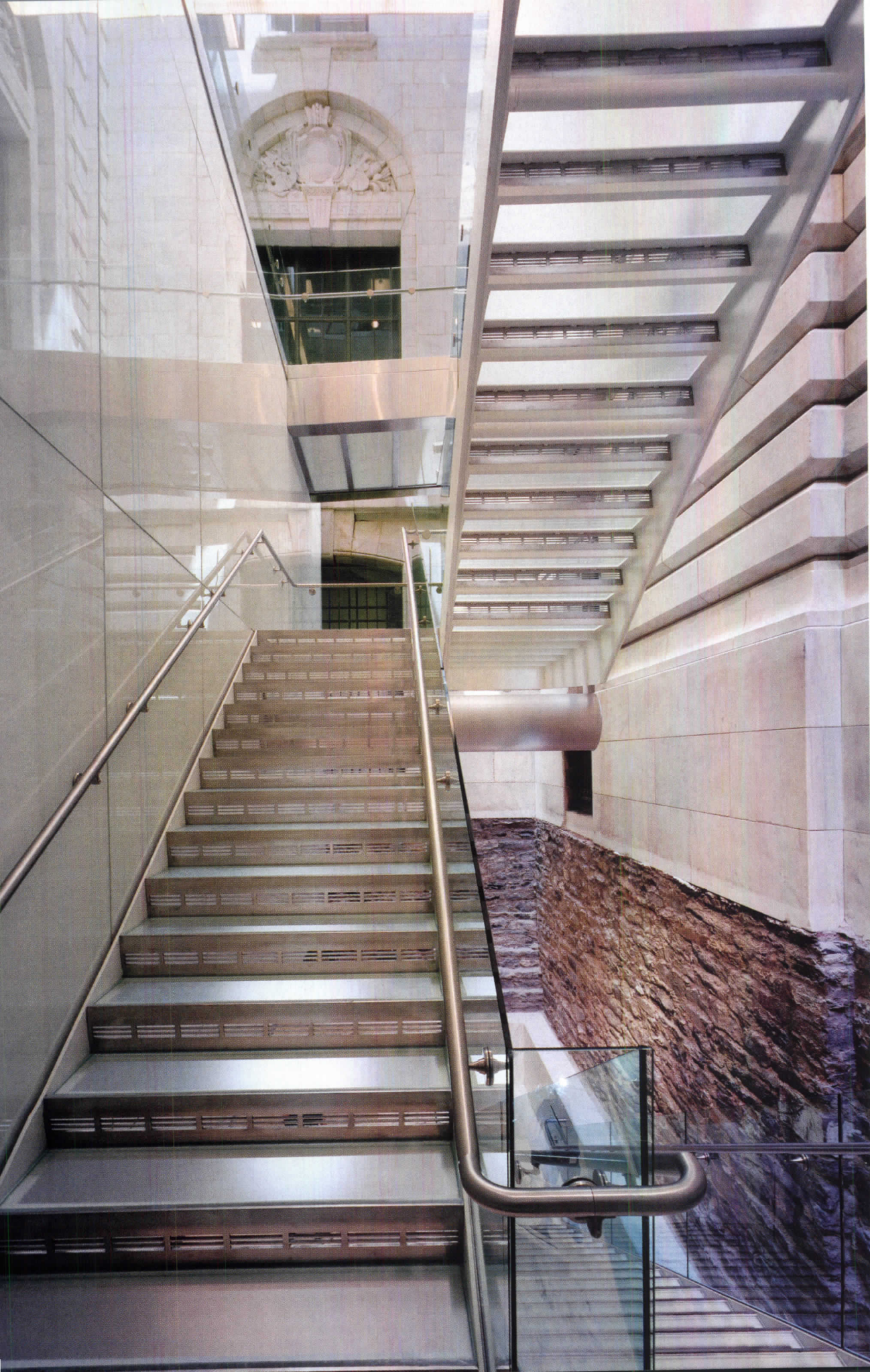
Directly beneath strip skylights, a structural-glass stair leads down two levels from the main floor to the auditorium (left), passing beneath the glass entry bridge (opposite, top).
