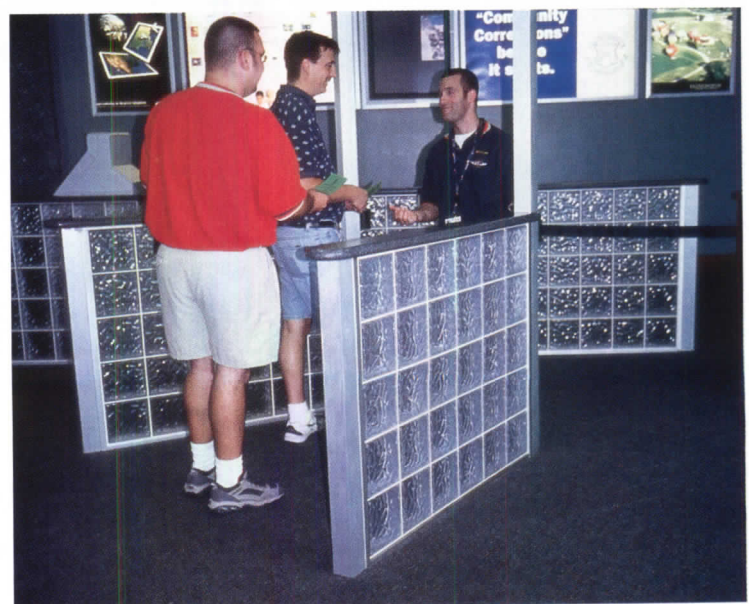
Waist-high acrylic block panels at the Southwest Airlines gate area at the Providence, RI airport help passengers line up for their flights.
