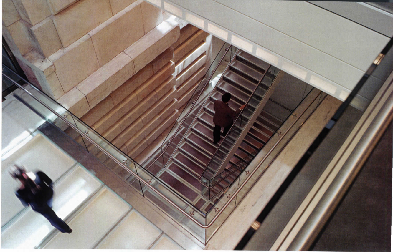
The stair descends past exposed rubble footings and terminates in a marble basin defined by new foundations (bottom left and right).
