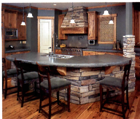
Concrete countertop mimics limestone.
