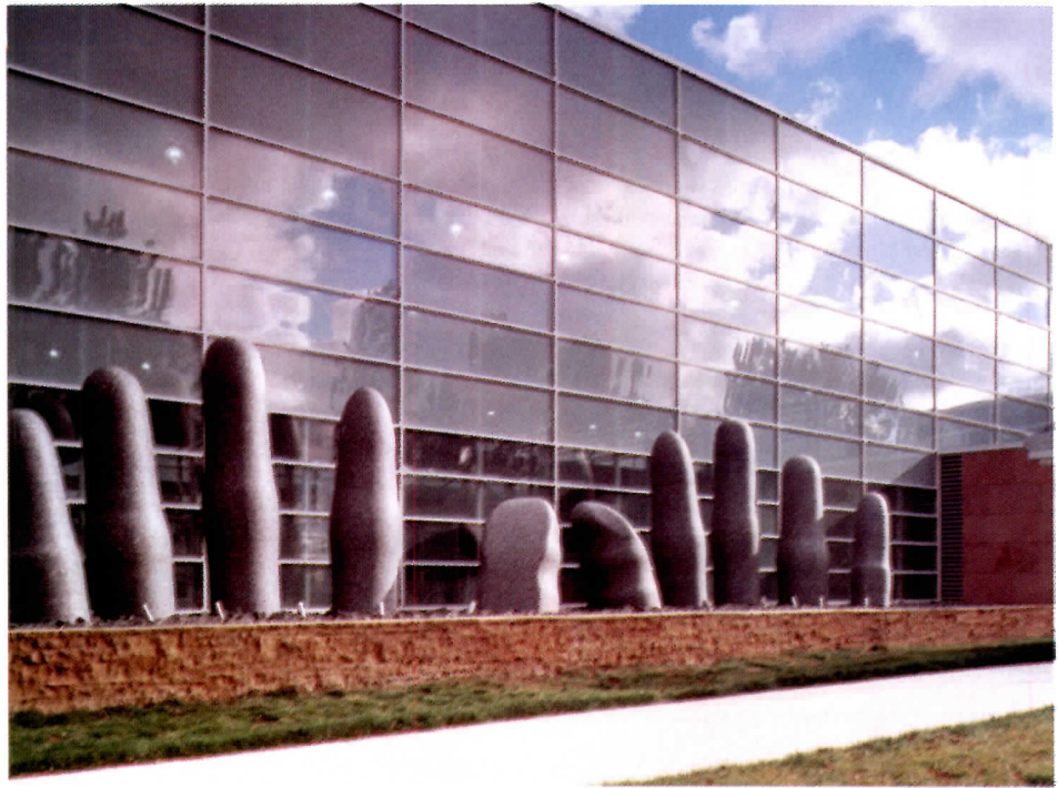
Ten granite fingers adorn the front entrance of the Phillips Plastics Custom Facility in Wisconsin.
