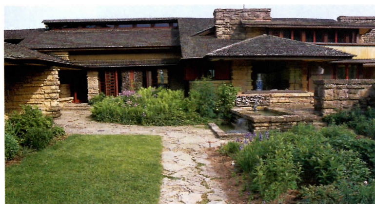
Wright built Taliesin on the side of a hill (top), which turns out to be a slippery slope. The house (above) needs as much as $60 million in renovation work.
