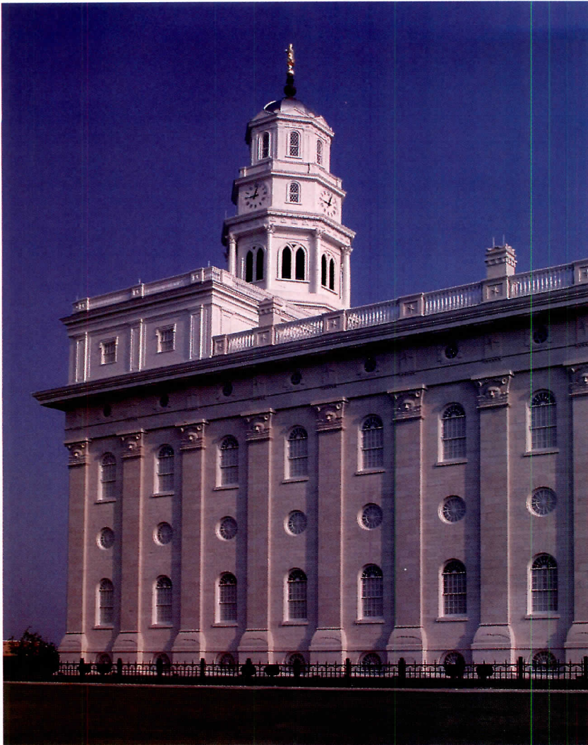
Nauvoo Temple in Illinois features hand-tooled and intricately carved limestone in six different finishes.
