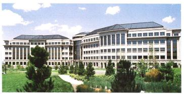
The all-precast structural systems for Starz Encore Headquarters, Englewood, CO includes double tees, inverted tee beams, shear walls and loadbearing precast walls. The system is a common approach to design in the Rocky Mountain region.
