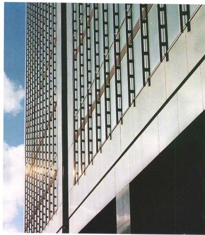
facade was fully engineered before bidding the job, in order to stress the high level of craftsmanship to the bidders. The German curtain-wall fabricator Seele GmbH won the bid with a proposal for a modified unitized system. "Other bidders' proposals were for more of a standard system approach, with room perhaps for some customization," says Carlos
