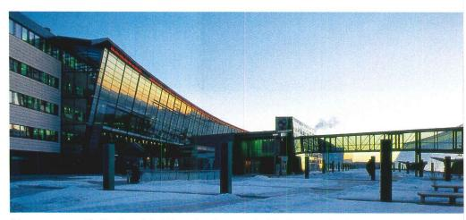
A long, narrow profile like that of the Telenor headquarters building is a common feature of sustainable design. If the building is oriented in the right direction, this form allows natural light to fall deep into the interior. Telenor says there is only about one lightbulb used per employee at Fornebu.
