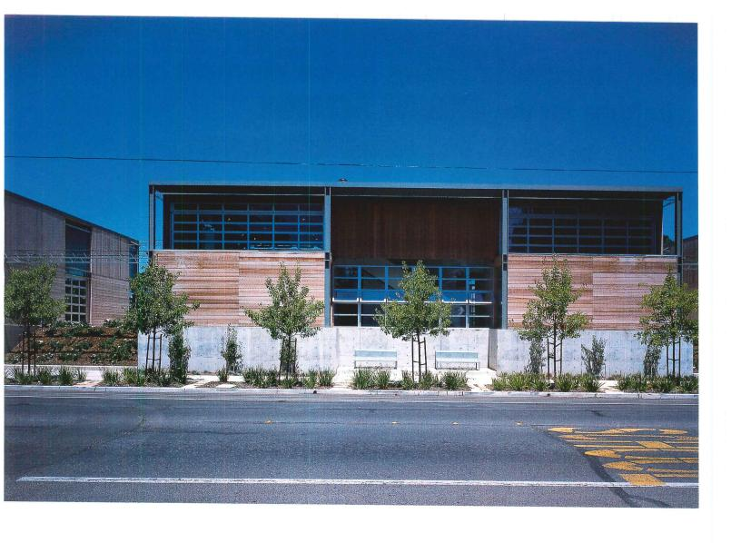
The new studio buildings (above and right) establish a formal but engaging street edge and provide spaces for street furniture, such as benches. Deep roof overhangs and limited fenestration on the lower portions of the buildings protect the south-facing elevations from the sun.
