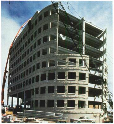
The architectural precast walls of 198 Inverness Drive West, Englewood, CO are the perimeter structural-gravity support for the floors and roof. Architect: POUW & Associates, Inc.
