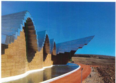
Calatrava designed the building so its rolling roof is assembled from straight wood members (above and left). The long load-bearing walls on the north and south also undulate, but they run parallel to each other, so roof beams remain the same size, except at the central bay. The east and west sides of the building are clad in corrugated aluminum (opposite, top).
