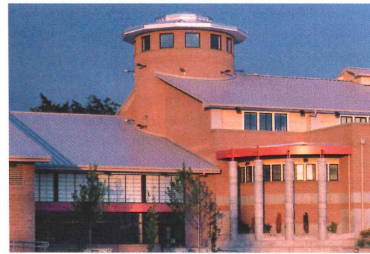
Masonry is often the sensible choice for schools, offering versatility, performance, affordability and easy maintenance—not to mention style. At North Whidbey Middle School Oak Harbor, Wash., sun plays off the school exterior enhancing its rich colors. Architects: DLR Group. Photo by Chris J. Robert
