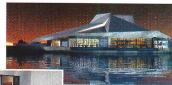
Tempe's Center for the Arts will include two theaters, a gallery, and a multipurpose room.
