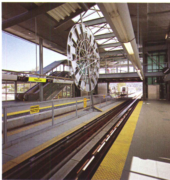
Columns branch into cantilevers to support twin, arching canopies (above). A second,
