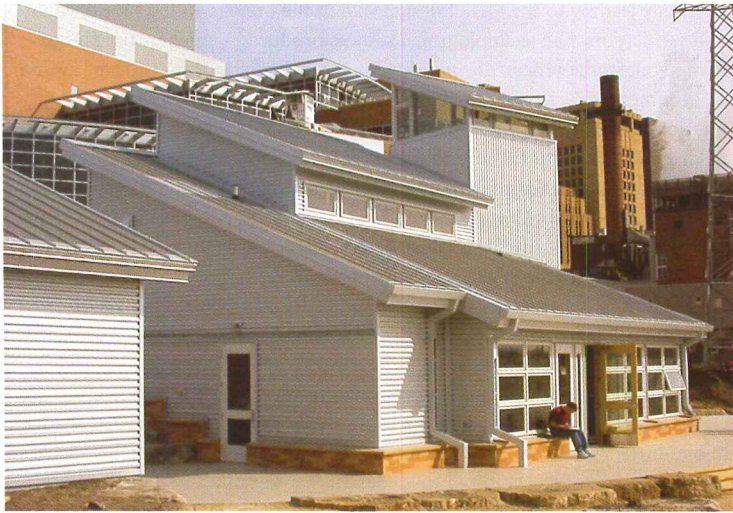
The Environmental Experiment Center (EEC) at the Science Museum of Minnesota in St. Paul followed a sustainable-design strategy and incorporates integrated energy-conserving technologies.
