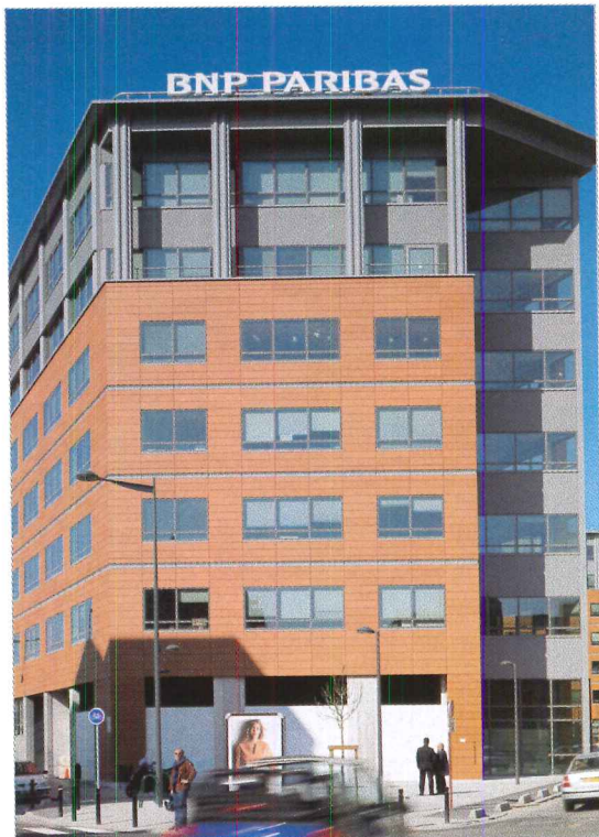
BNP PARIBAS Bank Building, Montreuil-Paris, France Architects: Arte Charpentier et Associés
