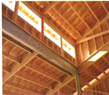
Clerestory windows help provide balanced day lighting. Environmental Experiment Center (EEC) at the Science Museum of Minnesota in St. Paul.
