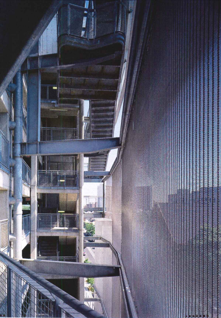
Stairs and ramps pulled away from the bulk of the 765-car garage work with metal mesh and glass
