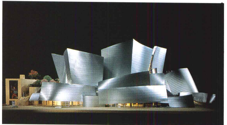
Design progress variation considered in limestone, 1992 (top). Final design model after switch to metal, 1998 (bottom).
