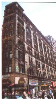
The Corbin Building in Lower Manhattan.
