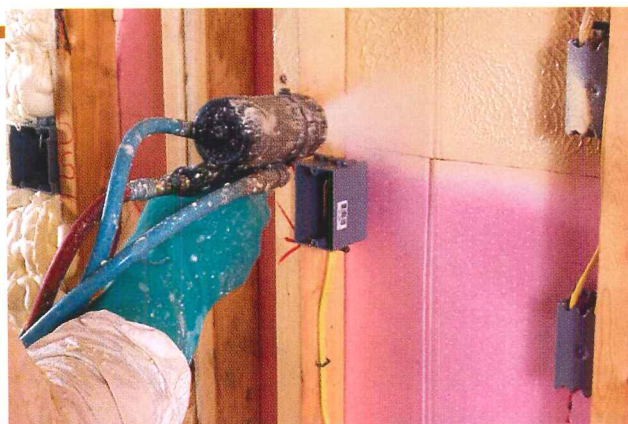
BioBase 501 is a low-density, open-cell-polyurethane, spray-foam insulation derived in part from soybean oil. Bio-Based Systems, Spring Valley, Ill. www.biobased.net CIRCLE 201
