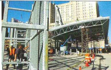
Workers completing WTC Path station.
