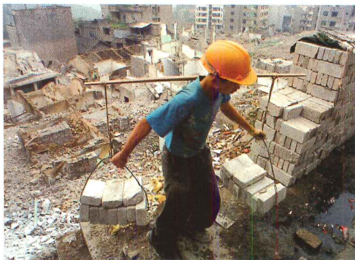
A worker removed pieces of old Wushan.
