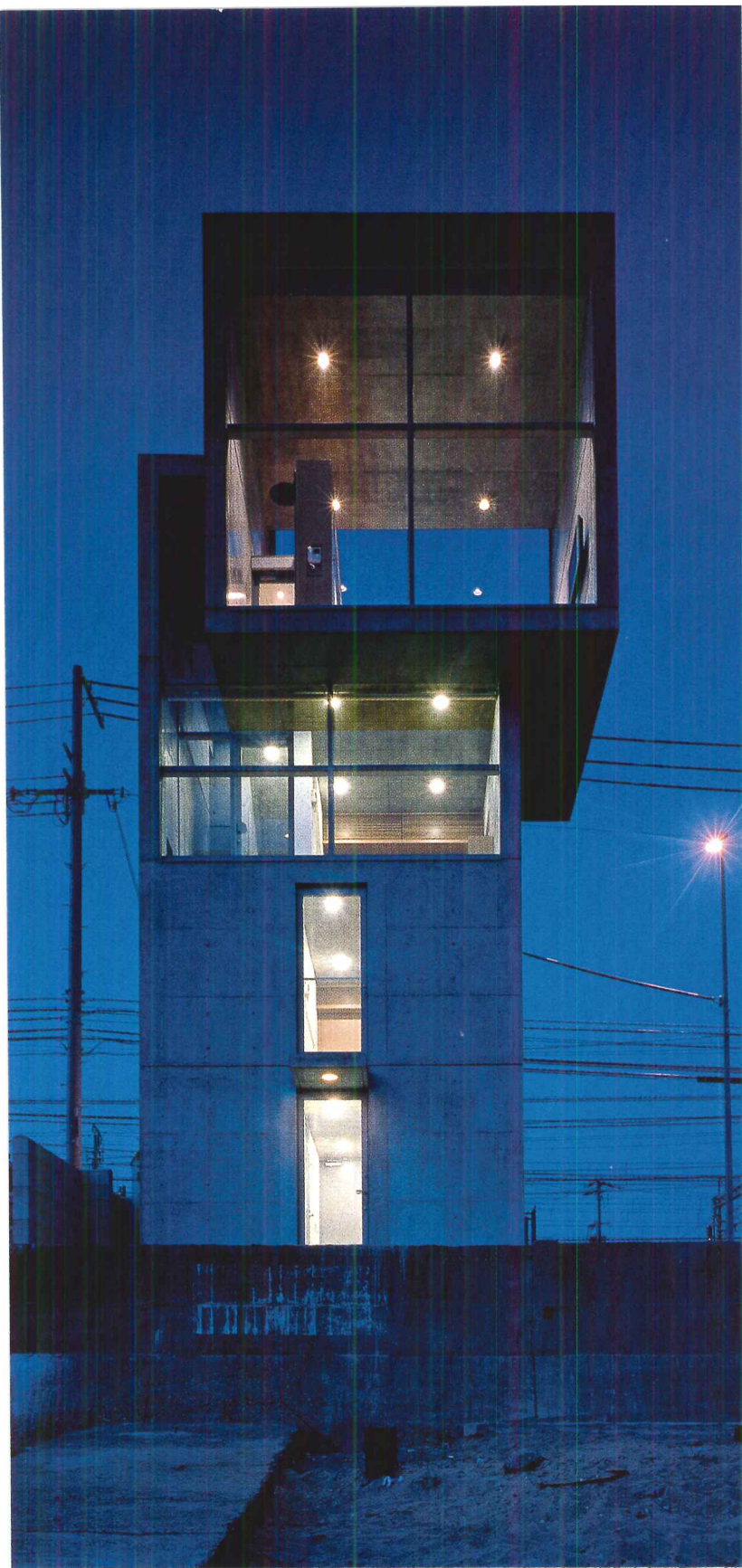
The architect plays his tower against the form and scale of the Akashi Strait Bridge (opposite, bottom). From inside the building's crowning cubic room (opposite, top), expansive views of bridge, sky, and city appear at once—in multiple directions. At night, when lit from within, the house reads as glowing volumes (above).
