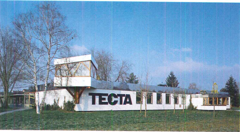
The existing 1960s concrete building now features various accretions, including the glass-and-wood lookout (bottom, left), with its expressively timber-framed panoramic window (bottom, right).
