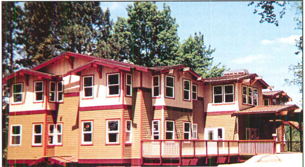
Oatfield Estates Extended Family Residences in Milwaukie, Oregon, is a fully wired retirement village. Each residence has a programmable logic controller (PLC), which automates appliances, HVAC systems, and even monitors the occupants.
