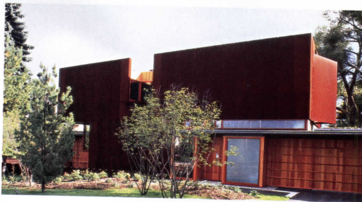
A strong urban face of Cor-Ten steel addresses the street on the north side of the house (above),
