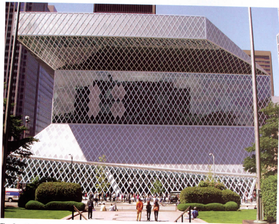
The Seattle Central Library has a sophisticated curtain wall, which was pre-engineered off-site.
