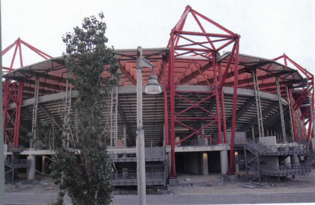
Braces supported the Karaiskaki Stadium in June.
