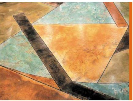
As the durability and cost-effectiveness of concrete make it increasingly popular for interior floors, architects are looking for ways to upgrade its appearance. Chemically reactive stains can be used to color newly cured concrete or to rehabilitate and update existing slabs. Courtesy L. M. Scofield.
