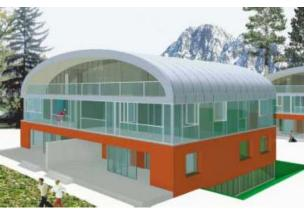
himmelrain, Sissach, Switzerland, 2004. These tri-level apartment buildings will be clad in varied materials, including plaster, glass, and zinc. The facades will have the effect of reducing the scale of the buildings to better integrate with the landscape.
