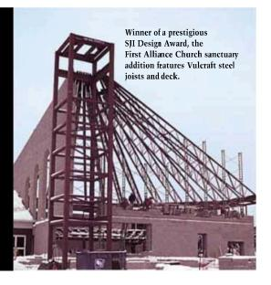
Steel joists also created greater headroom throughout the building by allowing both the catwalk and mechanical, electrical and plumbing systems to exist inside the structural envelope.
