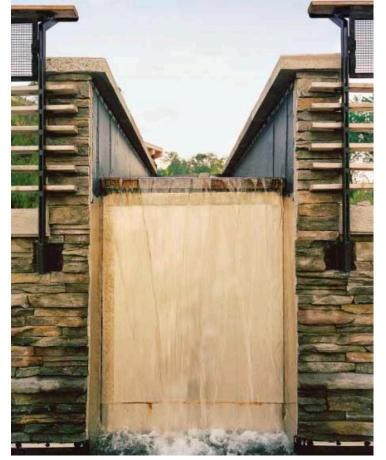
At the Discovery Health Center, rainwater flows into a trough (above), which is both an irrigation system and a holding tank for the fire-suppression system.
