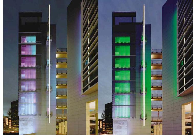
Metal-halide lamps illuminate the light tube (above two) used as a symbol of the oncecommon broadcast antenna. In the atrium, backlit stringers (right) make stairs appear to
