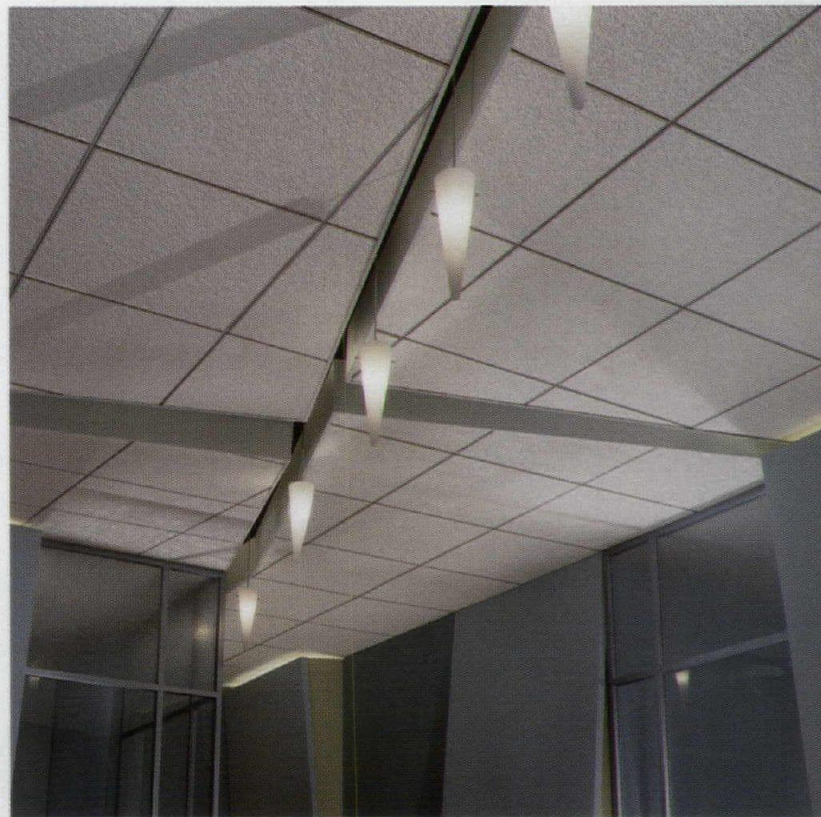
Many acoustical ceiling panels are made from mineral wool, gypsum and smaller amounts of paper and starch, as well as other miscellaneous materials. The mineral wool is made from slag, a by-product of steel manufacturing that consists of calcium silicate and other impurities.
