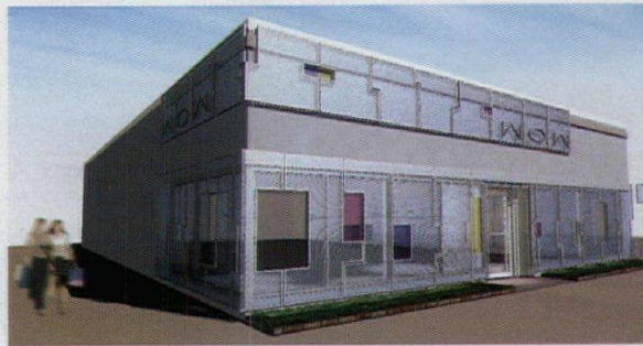
W.O.W., Newton, Mass., 2004 Experimentation with prototypes and materials resulted in a jigsaw-puzzlelike design for the building's facade. The store owners will be able to display their work in the apertures within the design.
