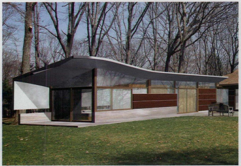
A complex, folded-roof structure (left) may top a suburban prototype Nastasi's firm has designed (above), which would be made of CNC-filled foam and glass-reinforced fiber.
