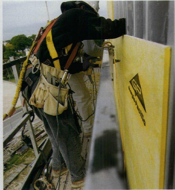
Georgia Pacific's DensGlass Gold Exterior Guard, a paperless glass-matted panel, has become a popular choice for exterior sheathing because it eliminates paper, a source for mold if the material gets wet during construction.
