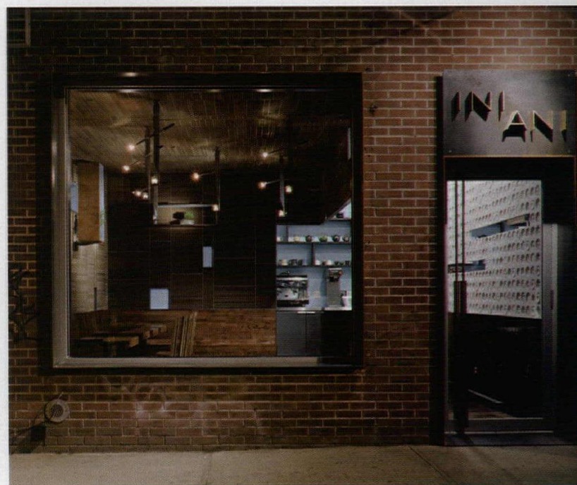
LTL opened up the entry (below) with generous glazing and built a box inside a box for the café (above).
