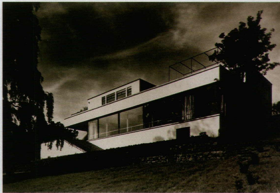
Mies's Tugendhat House in Brno, Czech Republic, remains a classic after 74 years.
