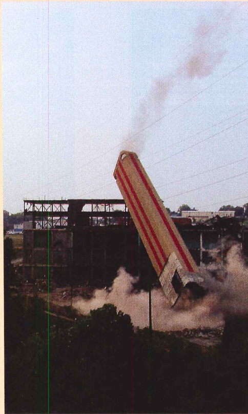
demolition. Electrical equipment from other parts was auctioned off as part of the demolition and dismantling of the entire complex.
