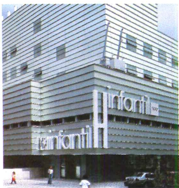
Gregorio Marañón Maternity and Pediatrics Hospital Madrid; Photography: © Duccio Malagamba
