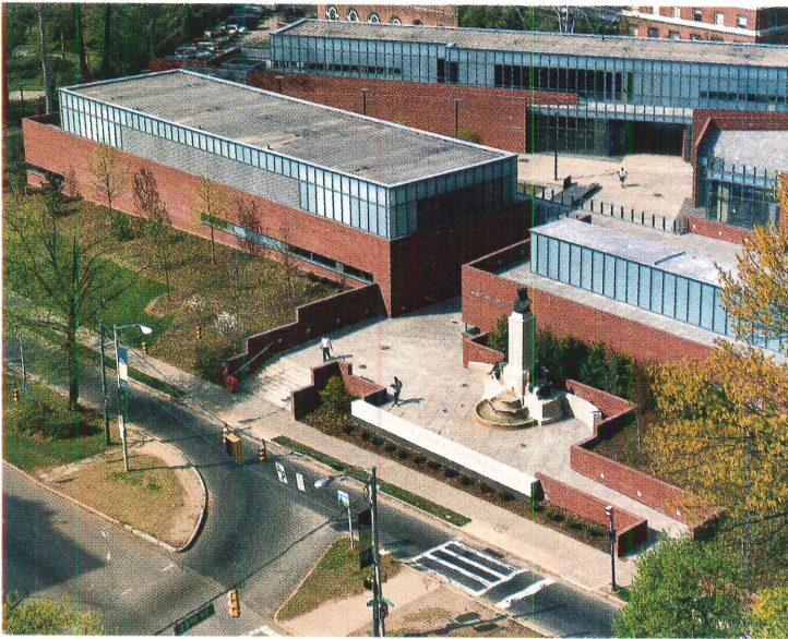
1. Smith Campus Center, Pomona College, Claremont, California Robert A.M. Stern Architects
