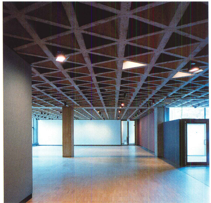
The Polshek Partnership is restoring Louis Kahn's Yale University Art Gallery with the kind of care that is usually reserved for antiquities. This photo shows one of the galleries as it was before work began.
