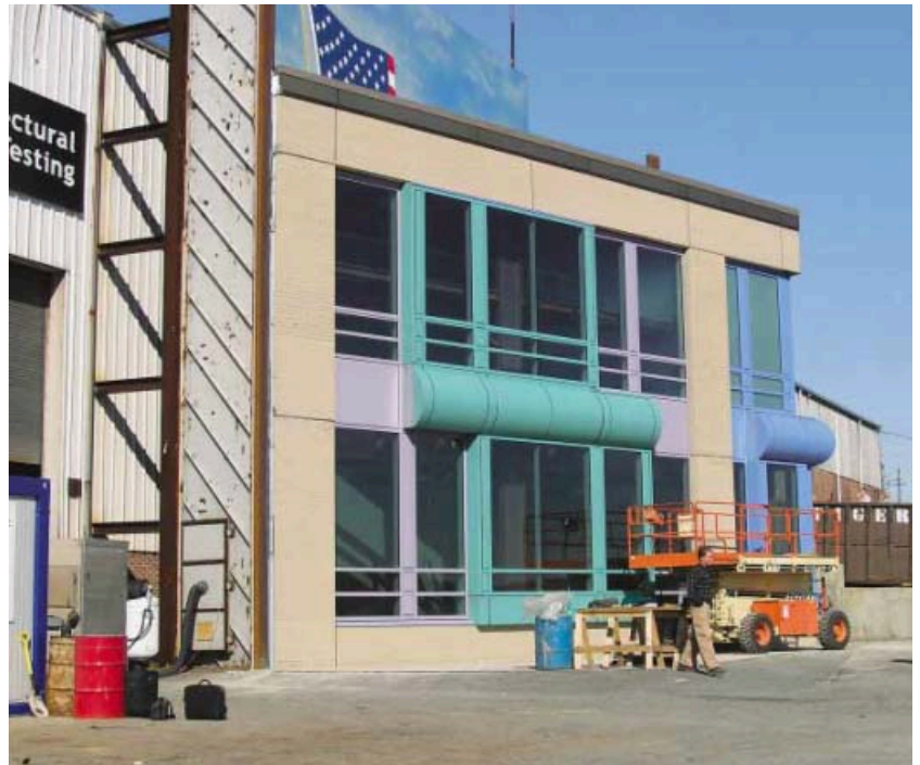
A battery of tests was conducted on a mock-up for the exterior lab wall of the Children's Hospital of Milwaukee, designed by Shepley Bulfinch Richardson and Abbott.
