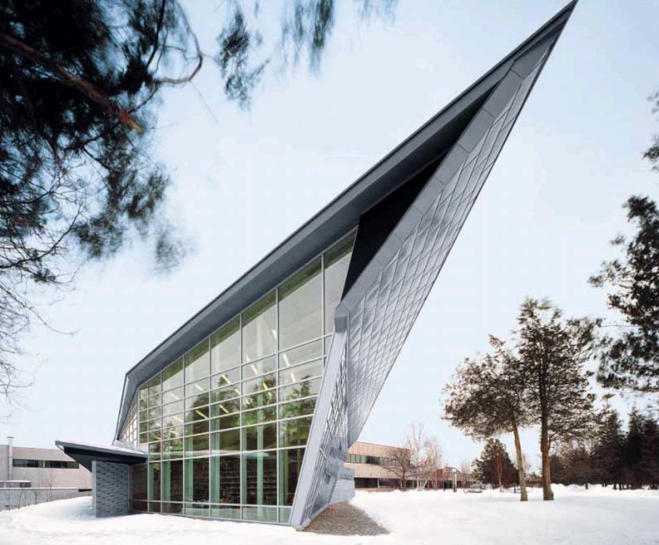
Loyalist College, Belleville, Ontario, Canada; Architect: Stephen Teeple Architects, Toronto, Ontario, Canada; Flat Lock Interlocking Wall Tiles; Fabrication and Installation: Simple Gooder, Toronto, Ontario, Canada
