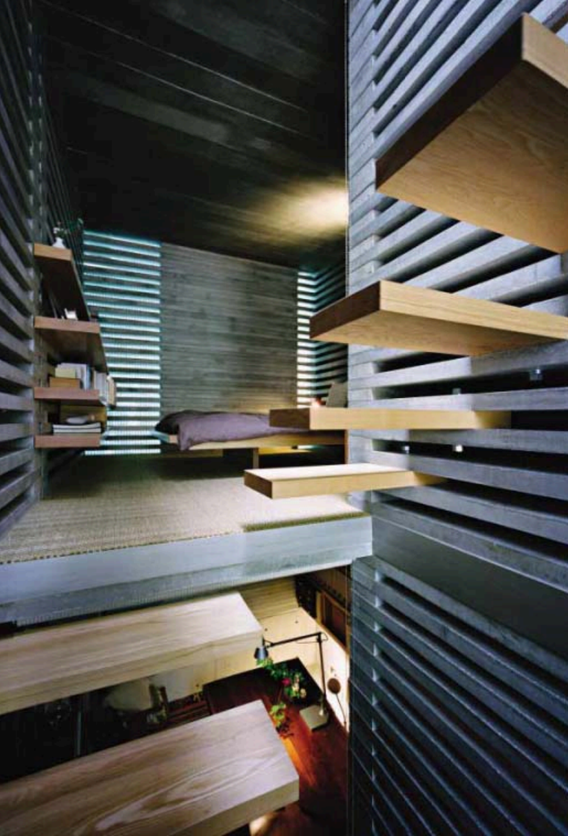
In the bedroom (left) and cavelike study (right), shelves of the same ash wood as the stairs cantilever from spaces between the concrete beams.
