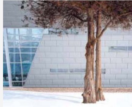
Loyalist College, Belleville, Ontario, Canada; Architect: Stephen Teeple Architects, Toronto, Ontario, Canada; Flat Lock Interlocking Wall Tiles; Fabrication and Installation: Simple Gooder, Toronto, Ontario, Canada
