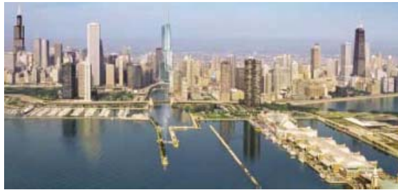
The tower (center) will dominate the city's waterfront.
