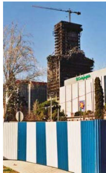
The tower's charred remains.
