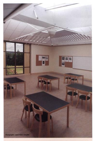
Mt. Angel high performance prototype classroom, Mt. Angel, OR: A rectangular suspended device dubbed "the halo" is made of translucent material that reflects part of the light onto the ceiling and walls, while letting part of the light into the room. Design team: BOORA, SOLARC, Prof. Charlie Brown of the Seattle Daylighting Lab, and SRG Partnership
