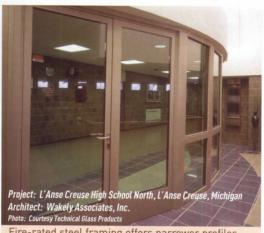
Fire-rated steel framing offers narrower profiles than traditional hollow metal steel frames.
