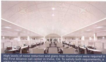
the First Alliance call center in Irvine, CA. To satisfy both requirements, a white non-woven acoustical fabric was attached to the top of perforated ceiling panels and back-lit to create a soft, luminous ceiling.
