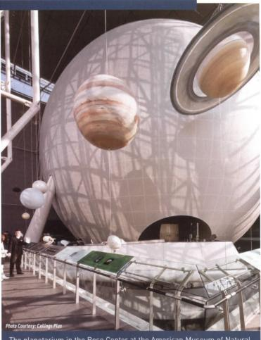
The planetarium in the Rose Center at the American Museum of Natural History, New York, established a benchmark for perforated acoustical panels. Designed by Polshek Partnership, the 87 ft. diameter sphere is clad with pearlescent metal panels and perforated to absorb noise in the resonant glass-box enclosure. Fabricating the precise compound curvature of the panels was only possible with recent advances in computer-assisted manufacturing.
