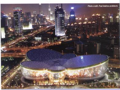
Shanghai Oriental Arts Center, Shanghai, China Metal mesh screens were laminated between structural interlayers to provide glare reduction and daylighting benefit. Architect: Aeroports de Paris, Paris
