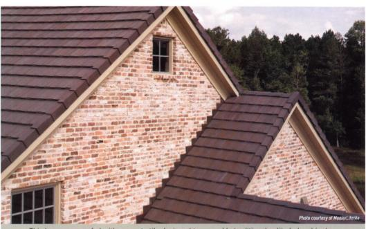
This home was roofed with concrete tile designed to resemble traditional split shake shingles.
