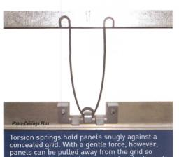
that the springs can be squeezed and released from the grid. Panels can then be removed or swung out of the way for maintenance.
