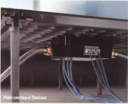
Modular wiring systems allow for improved management of power, voice, data and other wiring needs.
