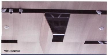
Even large perforated panels can be installed with torsion springs that allow panels to swing out of the way for above-ceiling maintenance. This photo from the Clinton Library also shows one way that lighting can be integrated into an attractive design.
