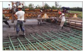
**Hycrete Admixture is** rated by MBDC as a biological nutrient. It converts concrete from a hydrophilic to a hydrophobic material, so that it repels water (right). It chemically bonds with steel to create a nonsoluble layer that coats reinforcing bars (above) and lodges in the capillaries of the concrete to block water passage.
