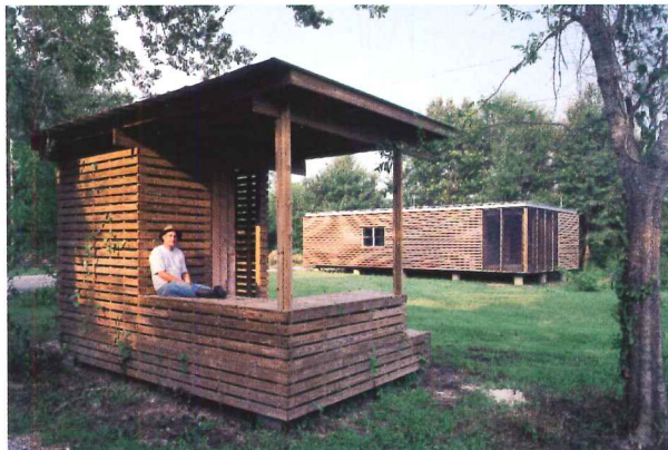
Frank's House, Masons Bend, Alabama: Second-year students still design and build houses; this one recalls a double-wide trailer.
