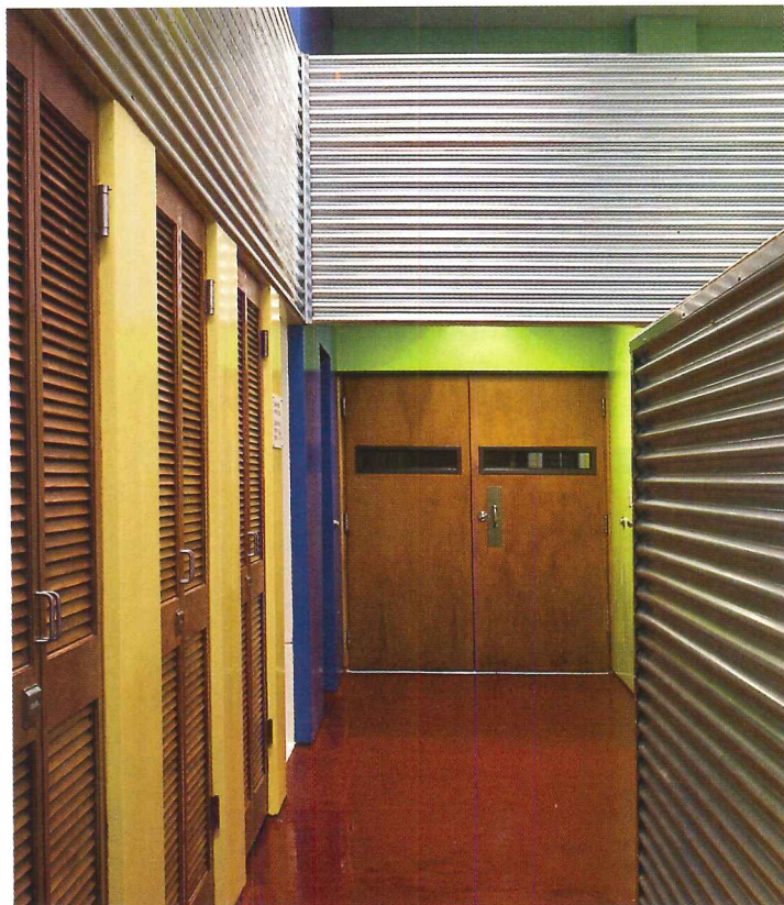
Fourteen-foot-long curtains in the massage and Pilates areas stand in for built partitions (above). Easy-to-maintain finishes in the dressing room area include an epoxy-resin floor, metal panels, and louvered doors (left).
