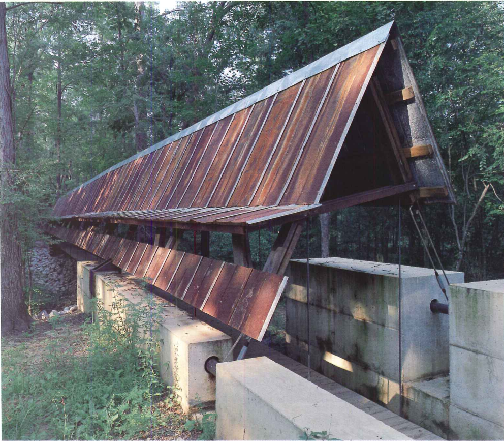
Bridge, Perry Lakes Park, Perry County, Alabama: This 140-foot-long metal-and-cypress-covered bridge crosses a swampy lake and provides pedestrian access to the east side of the park. Engineered by Robert McGlohn, the bridge has three triangular horizontal trusses and end sections stabilized by cables anchored in concrete.
