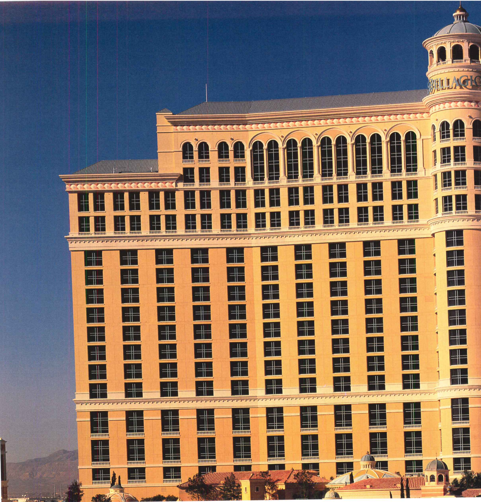
The Bellagio Las Vegas Photo courtesy of Dryvit Systems, Inc.
