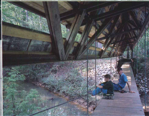
Bridge, Perry Lakes Park, Perry County, Alabama: This 140-foot-long metal-and-cypress-covered bridge crosses a swampy lake and provides pedestrian access to the east side of the park. Engineered by Robert McGlohn, the bridge has three triangular horizontal trusses and end sections stabilized by cables anchored in concrete.
