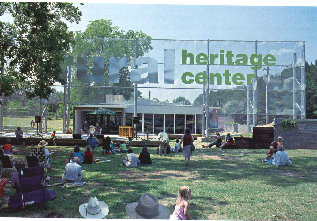
Rural Heritage Center, Thomaston, Alabama: The Rural Studio took an existing 1950s building, renovated it, and expanded it to create this new facility. A 100-foot-long sign made of perforated metal set on vertical trusses gives the building a civic presence and backdrop for an outdoor performance space.
