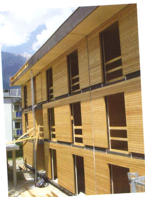
Clockwise from top left: An apartment complex in Innsbruck uses BBS panels for all structural walls. This spa in southern Austria uses the panels in the overhang. In the small project shown here, they are used as simple
