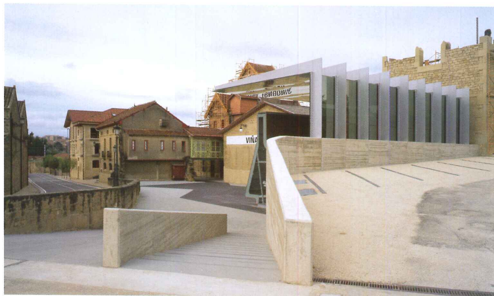
The steel-finned canopy for the pavilion abuts a retaining wall and a parking area in the villagelike winery.
