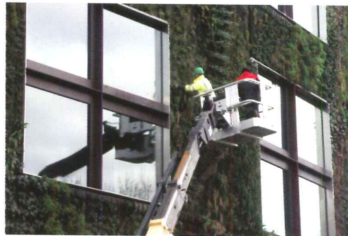
About 150 plant species are growing on one face of the Musée du Quai Branly, in Paris (left). Required maintenance, primarily trimming of overgrown plants, is conducted about three times a year.
