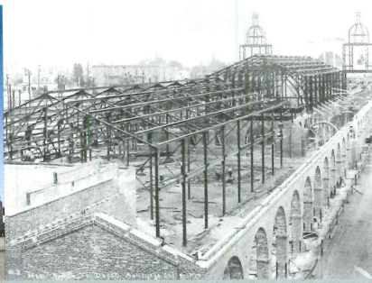
The Amtrak station, in the Santa Fe Depot; the Jacobs Building, a converted baggage building; and the Copley addition, viewed from the south (far left). A construction photo shows the depot's steel frame going up atop the arched concourse (near left).
