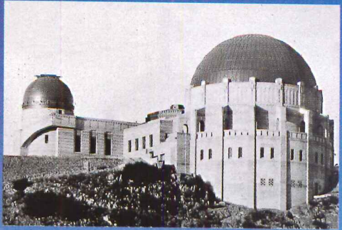
Architects John C. Austin, AIA, and Frederic M. Ashley, FAIA, considered the 1935 observatory design a "Modified Greek" style. Originally unfinished concrete, restoration architect Brenda Levin says it was most likely painted white in the 1940s to hide corrective patches and joints.
