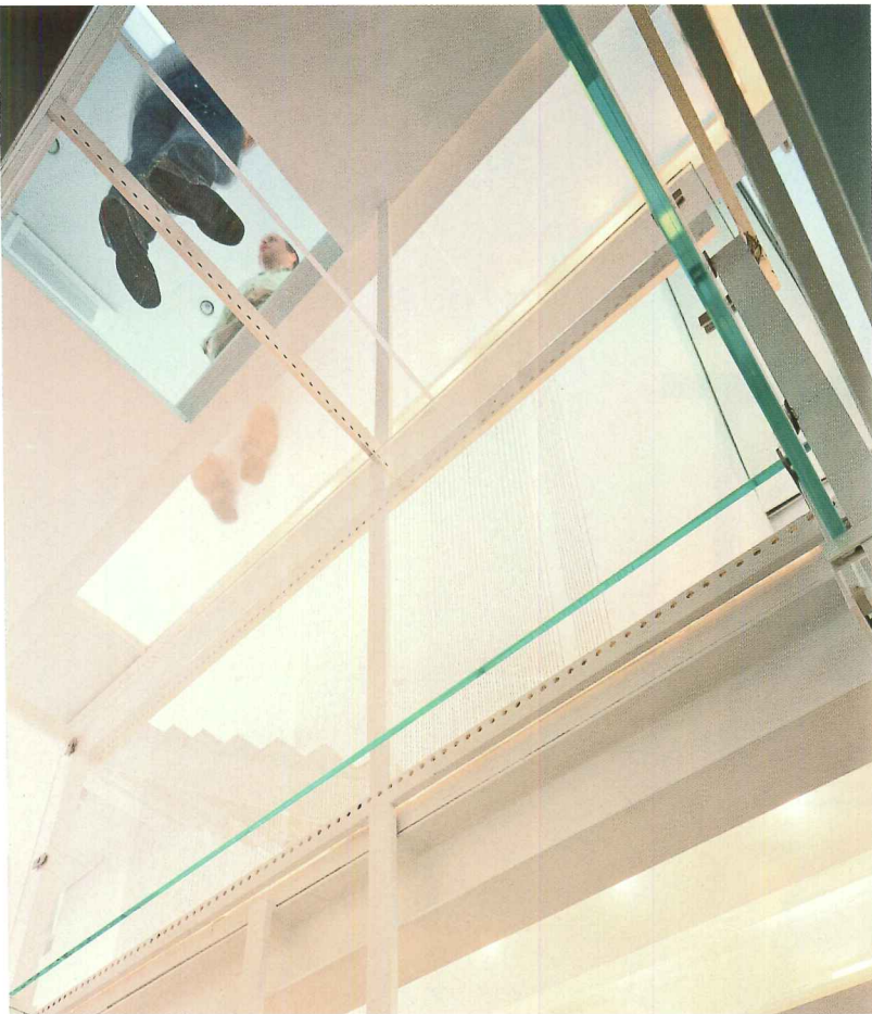
After removing a dumbwaiter, the architects sealed off the shaft with clear acrylic (left). They installed a new opaque-solid-surface master tub (below) in place of the original transparent one west of the master bedroom.
