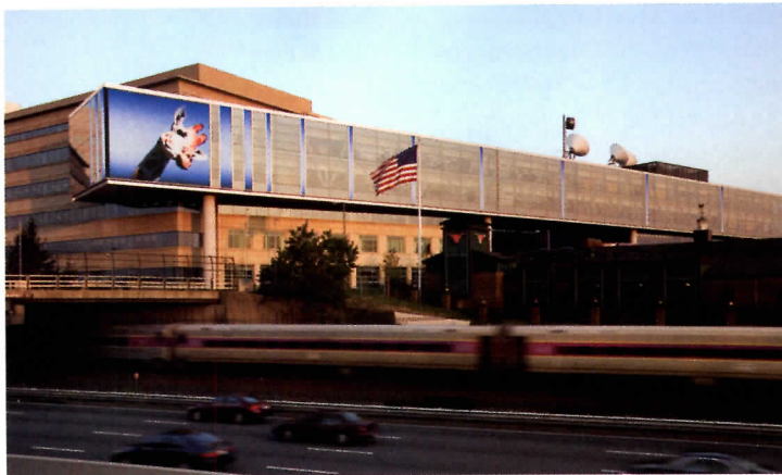
At WGBH, Polshek Partnership turned part of the facade into an LED mural.
