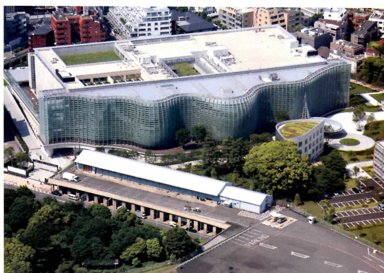
A billowing wall of aluminum and glass (opposite and above) creates an organic curtain between the outside and inside of the multilayered center. The precast-concrete box of exhibition space and the glazed public areas, nestled on a green site in the densely settled Rappongi district, are clearly defined (right).
