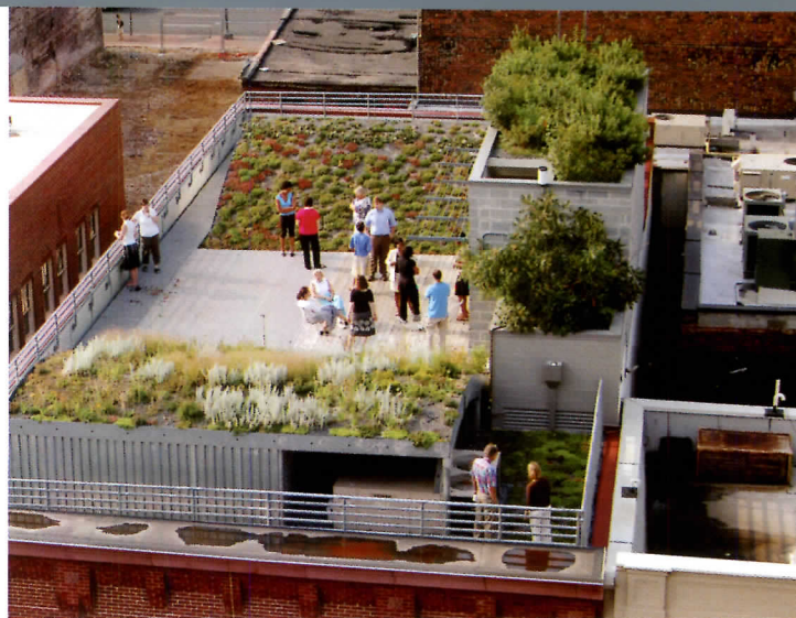
The installation includes planted "waves" that hide rooftop mechanical units.
