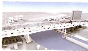
Only the pier designs (right) differ in two options for a new I-35W bridge (left).
