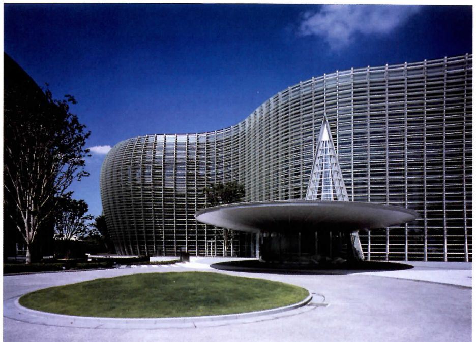
A billowing wall of aluminum and glass (opposite and above) creates an organic curtain between the outside and inside of the multilayered center. The precast-concrete box of exhibition space and the glazed public areas, nestled on a green site in the densely settled Rappongi district, are clearly defined (right).
