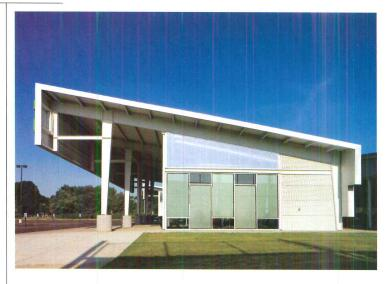
The architects folded a standing-seam metal roof (left and opposite, bottom) around the roof structure to provide shading. Throughout the night, bright lights signal a safe and secure environment (opposite, top).
