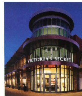
Victoria's Secret, Chino Hills, CA Architect: McCall Design Group Custom-engineered Storefront by Oldcastle Glass® Vistawall®
