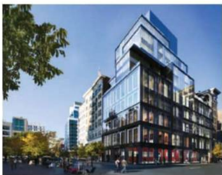
LEFT: 15 Union Square, the original home of Tiffany & Co., designed in the 1870s by John Kellum, was updated and its cast-iron structure revealed to create a harmonious partnership between historic and Modern.
