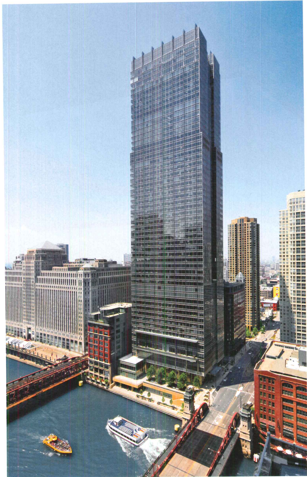
An articulated steel crown defines 300 North LaSalle on its prominent site. To maximize the southern exposure of the garden and limit solar gain on the east and west facades, the team placed the tower on the plot's northern limit.
