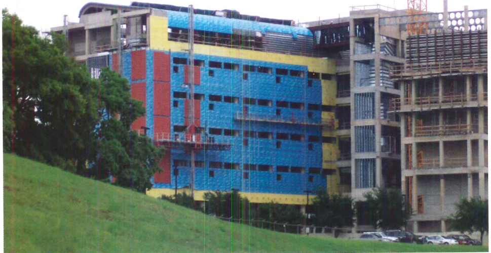
Air barriers with no mechanical fasteners are able to seamlessly wrap a structure for additional energy savings.
