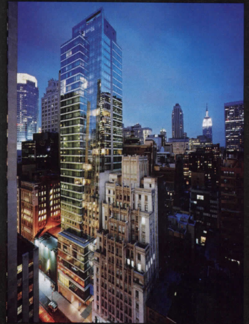
The Centria / 18 West 48th Street, NY Architect: Perkins Eastman
