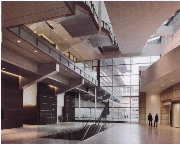
BRONX COUNTY HALL OF JUSTICE RAFAEL VIÑOLY ARCHITECTS 10. Displacement ventilation inside and a glazed curtain wall paired with interior light shelves are two of this building's sustainable strategies.
