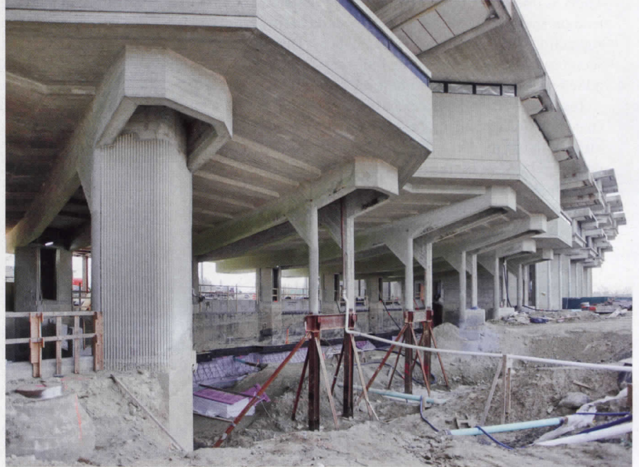
MAKING CONNECTIONS On the west side of the link, designLAB excavated around Rudolph's bulbous columns (right) and tucked the new facade under his projecting eaves (top). Stainless-steel screens help shade the glass addition. Above, the campus in 1985.
