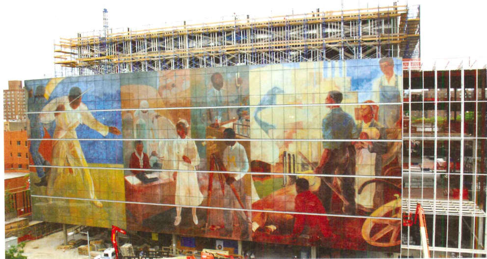
The curtain wall facade on the Harlem Hospital New Patient Pavilion features a digitally applied artistic mural that provides light control while still allowing vision out.
