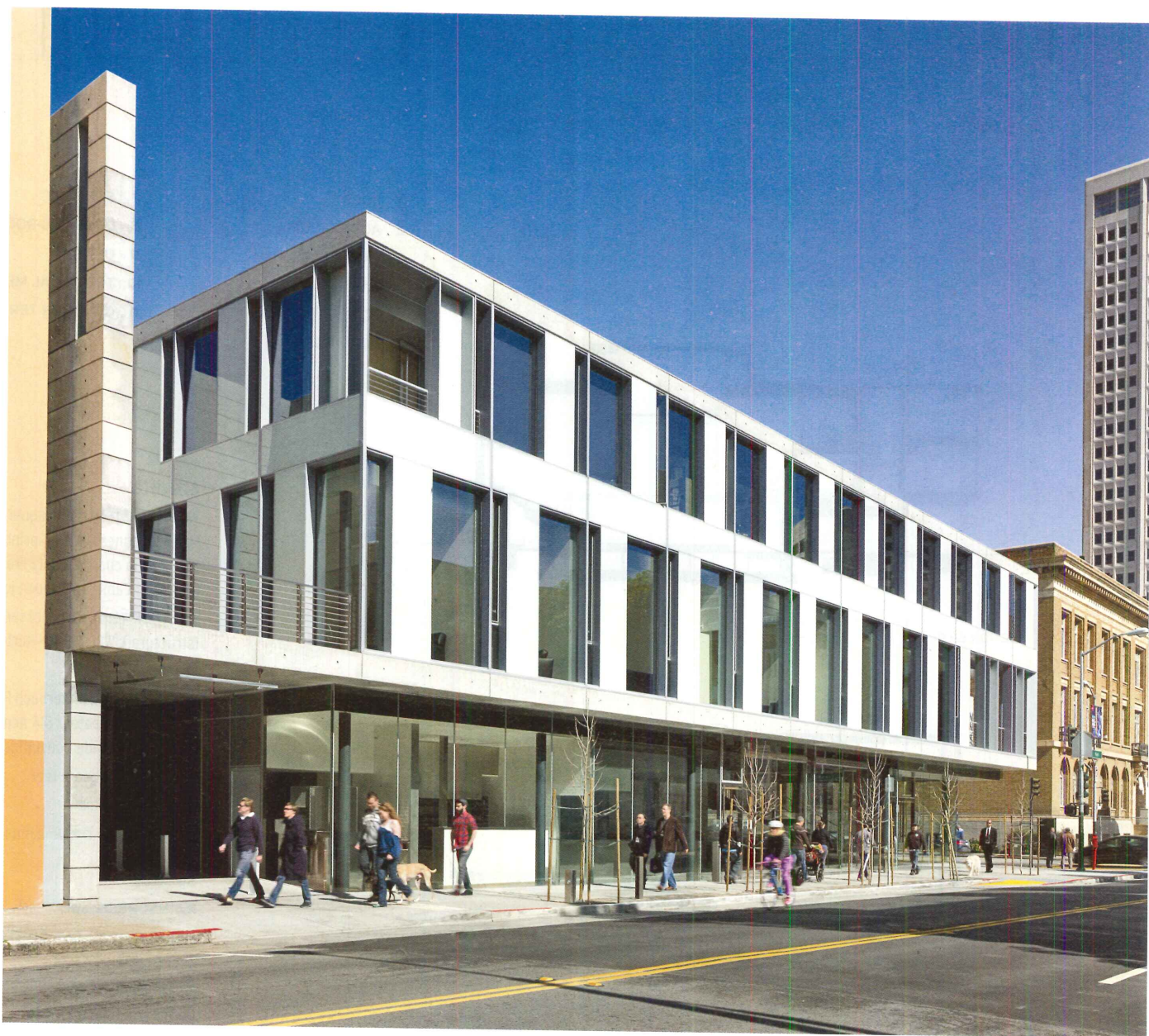
DISCREET TRANSPARENCY The architects pierced the poured-in-place-concrete structure with glass window walls so pedestrians standing outside the south facade (right) or the north facade (opposite) can observe activities within.
