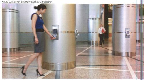
The addition of access-card readers to the user control panel allows customized service.
