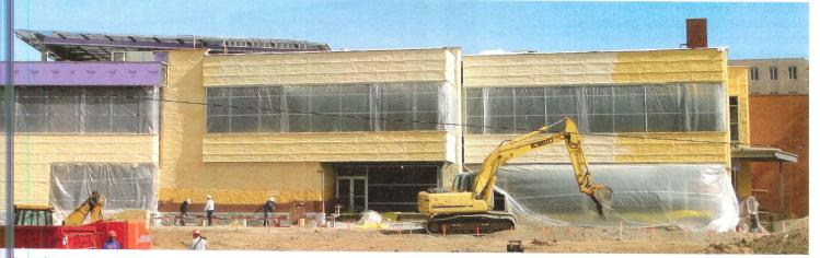
Me dium-density closed cell insulation can be spray applied to the outside of the sheathing on a stud cavity wall assembly and remain durable and war er resistant during the construction period.
