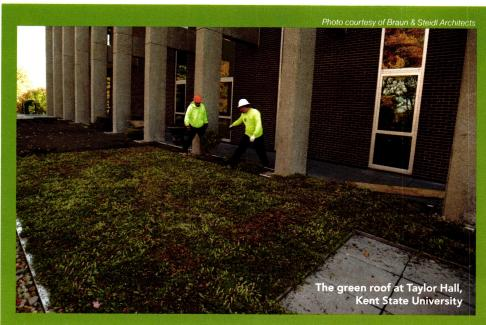
The benefits of green roof technology are wide ranging. They include management of stormwater, reduction of heat island effects, restoration of habitat, biodiversity of plant and wildlife, water efficiency, energy optimization through both cooling and heating, reuse of building materials, recycled-content materials, increased roof durability and longevity, and creation of rooftop amenity spaces.
