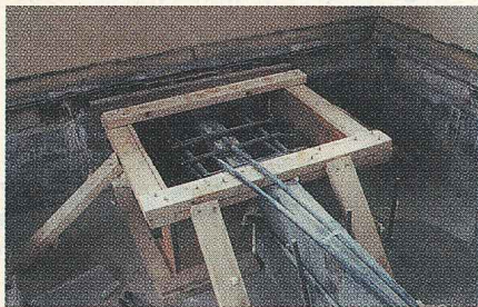
INSIDE JOB Post-tensioning of beams, to arrest up to 7 in. of sagging, raised cantilever less than 1 in.
