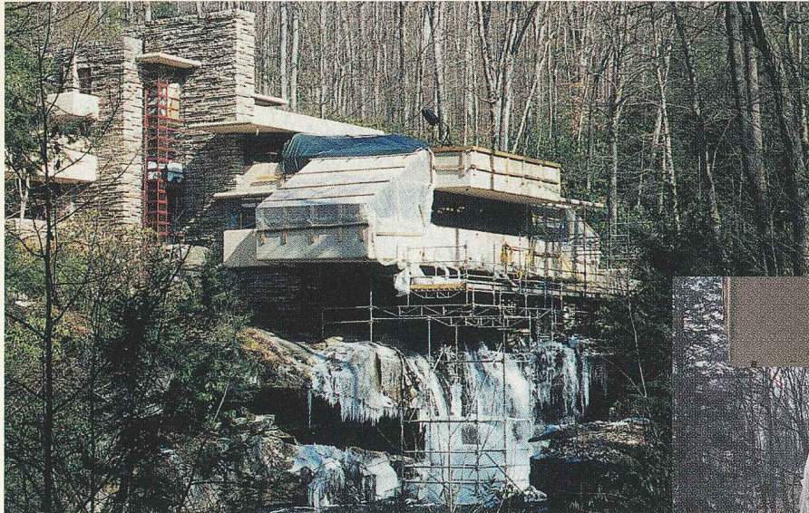
OVER WATER Fallingwater's cantilever, shored since 1997, gets fixed.
