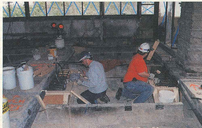
INSIDE JOB Post-tensioning of beams, to arrest up to 7 in. of sagging, raised cantilever less than 1 in.
