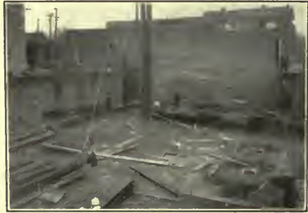
Dec. 15, 1902.—Excavation complete and column bases set.
