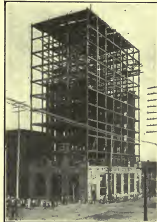
Feb. 15.—Limestone to height of second-story window sills. Roof tier of beams in place and fireproofing in six stories.
