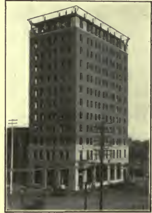
April 1.—Brickwork to lower tier of cornice.
