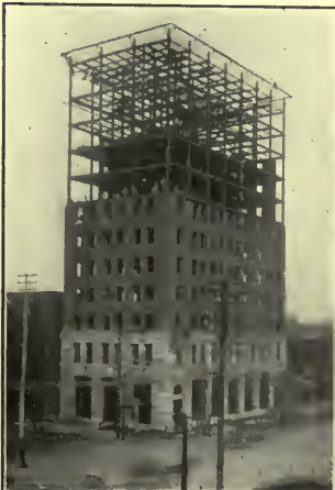
March 13.—Brickwork seven stories high.
