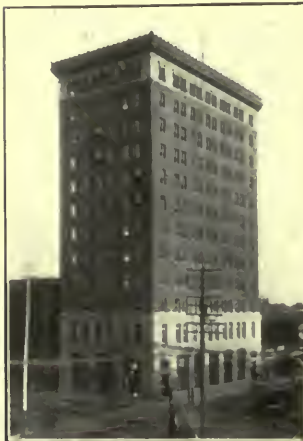
July 1.—External construction finished.
