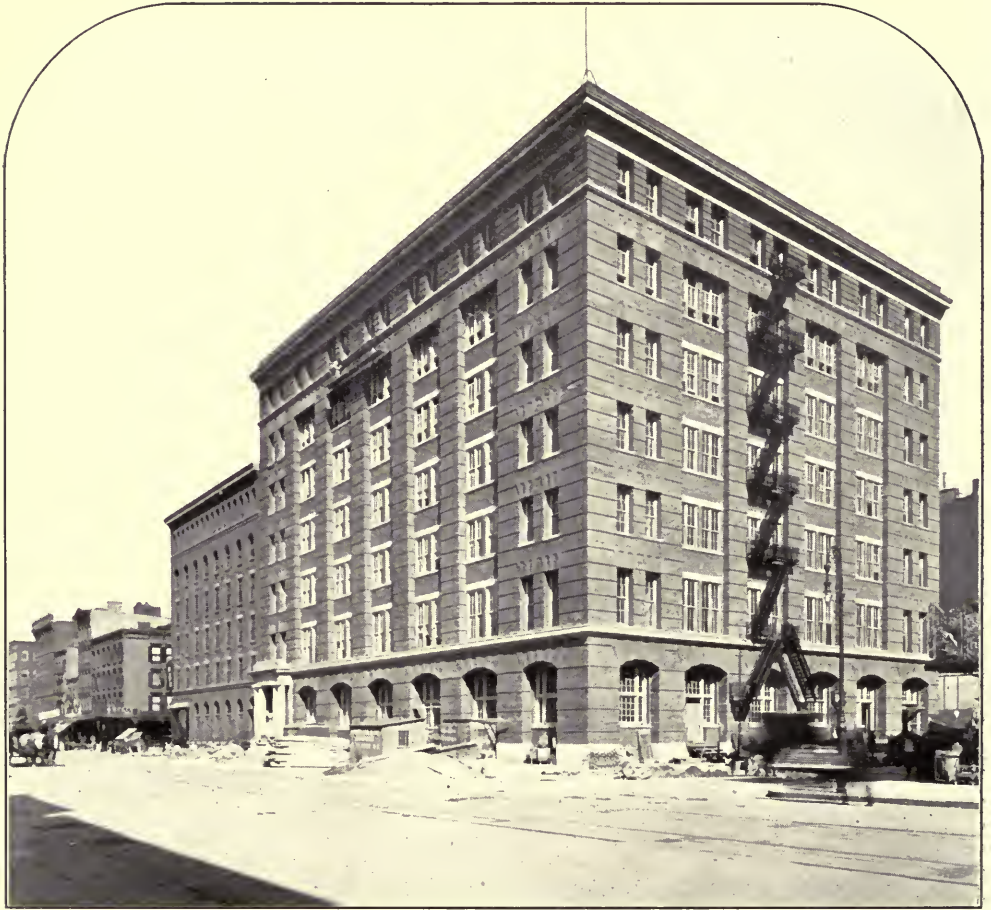
FIG. 1.—THE OXLEY-ENOS AND THE STREET & SMITH BUILDINGS.
