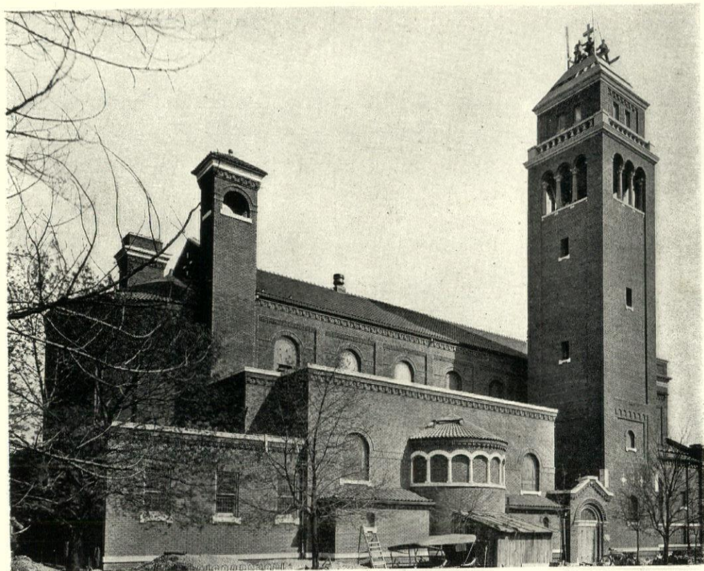
DETAIL OF WEST AISLE—HOLY ROSARY CHURCH, DAYTON, OHIO. W. L. Jaekle, Architect.
