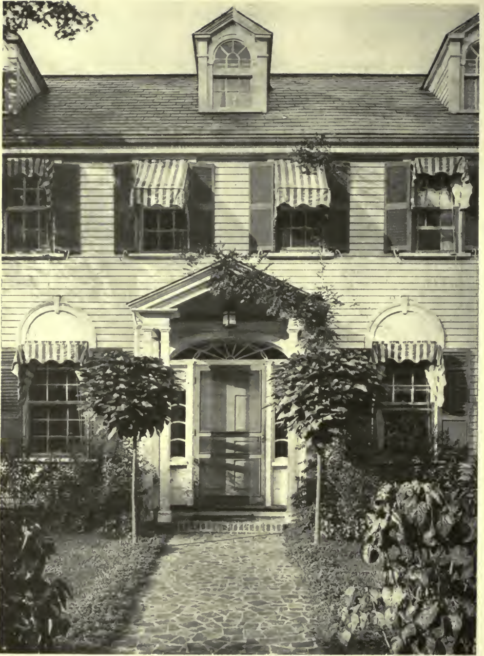
DOOR DETAIL—RESIDENCE OF W. N. HARTSHORN, ESQ., CAMBRIDGE, MASS. GRANDGENT & ELWELL, ARCHITECTS.
