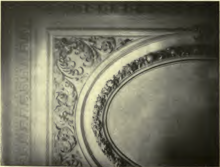
STAIRCASE CEILING—THE PYNES.
