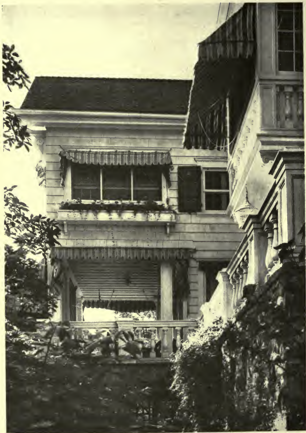
RESIDENCE OF WALTER CRITTENDEN, ESQ., CORNWALL-ON-HUDSON, N. Y. PARKER MORSE HOOPER, ARCHITECT.
