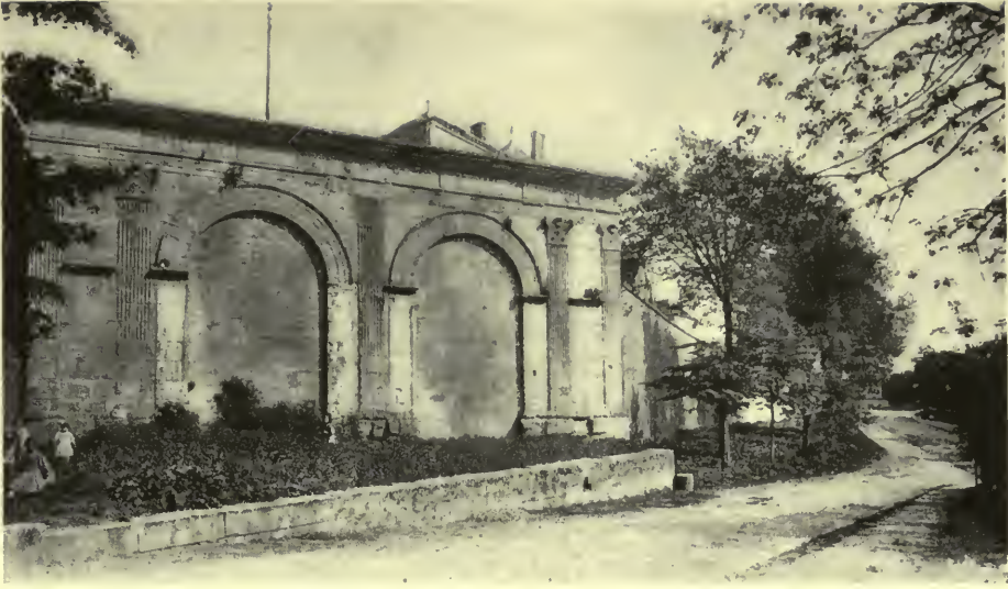
REMAINS OF ROMAN GATE AT LANGRES.
