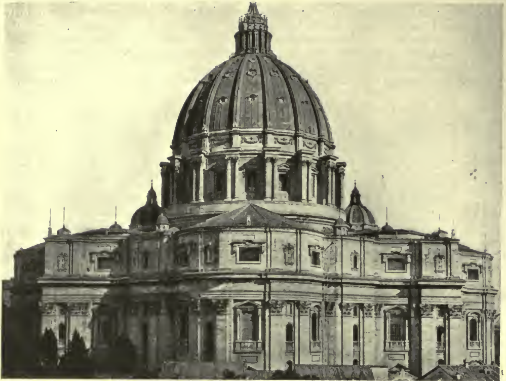
DRUM OF ST. PETER'S. BUTTRESSES OF DRUM PRODUCE SATISFACTORY EXPRESSION OF STABILITY.
