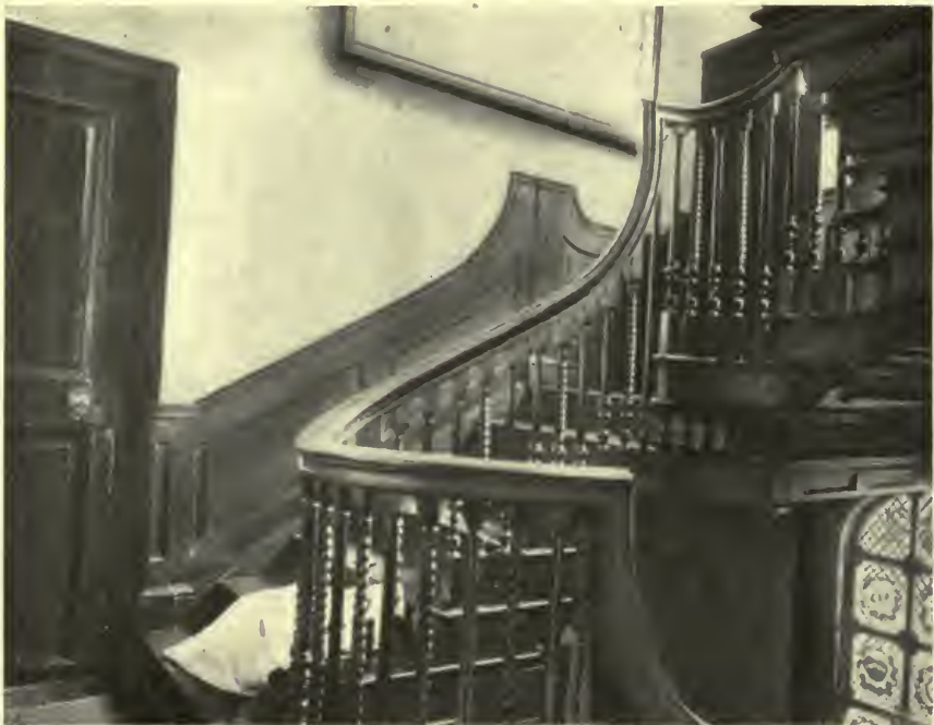
STAIRCASE—UNLAWATER, NEWNHAM-ON-SEVERN, GLOUCESTERSHIRE.
