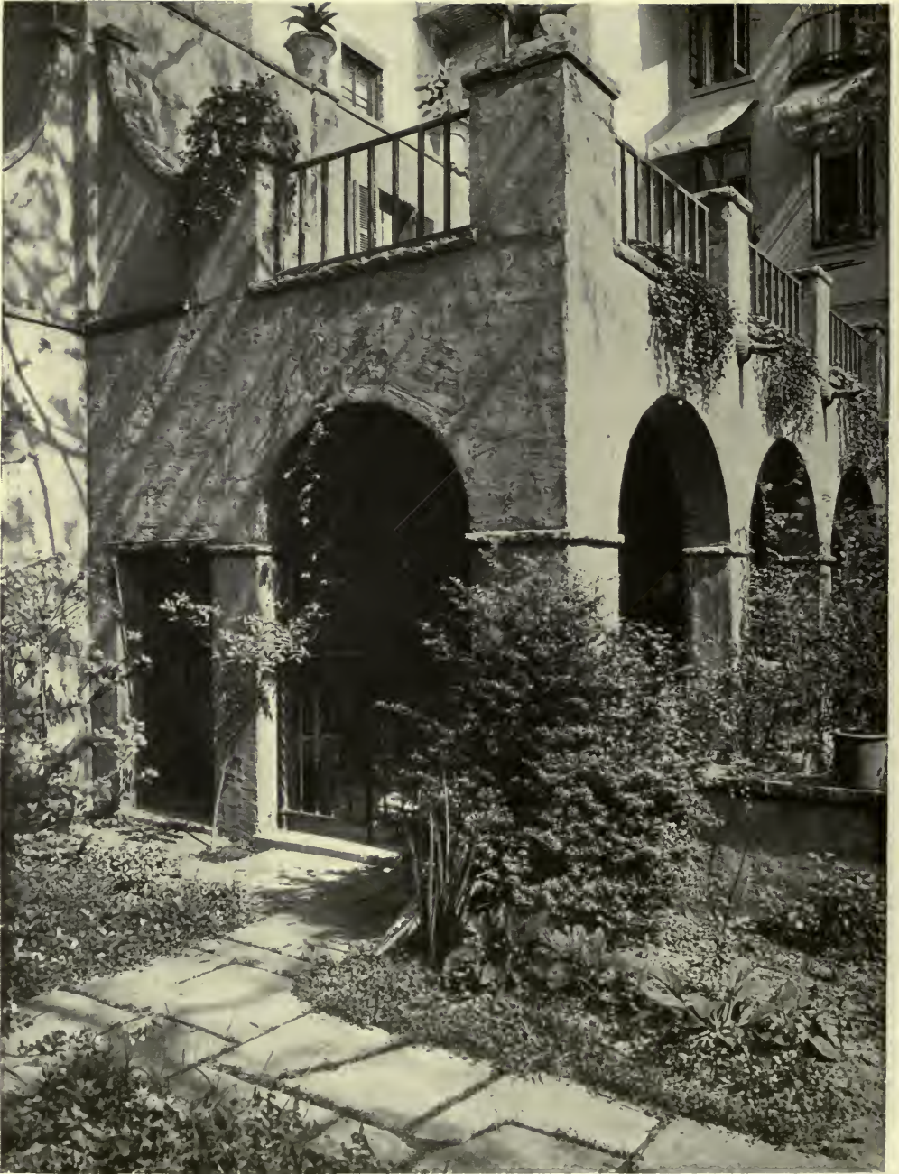
LOGGIA AT REAR OF ONE OF THE FORTY-NINTH STREET HOMES—TURTLE BAY GARDENS, NEW YORK CITY. EDWARD C. DEAN AND WILLIAM LAWRENCE BOTTOMLEY, ASSOCIATE ARCHITECTS.
