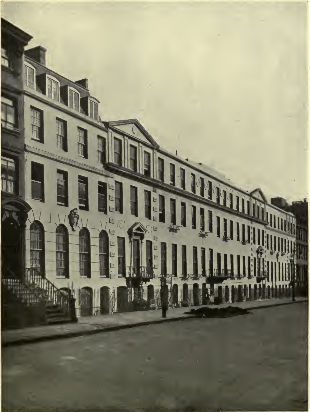
FORTY-EIGHTH STREET FAÇADE—TURTLE BAY GARDENS, NEW YORK CITY. EDWARD C. DEAN AND WILLIAM LAWRENCE BOTTOMLEY, ASSOCIATE ARCHITECTS.
