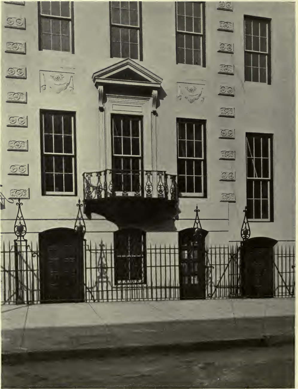
DETAIL OF ONE OF THE FORTY-EIGHTH STREET HOUSES—TURTLE BAY GARDENS, NEW YORK CITY. EDWARD C. DEAN AND WILLIAM LAWRENCE BOTTOMLEY, ASSOCIATE ARCHITECTS.
