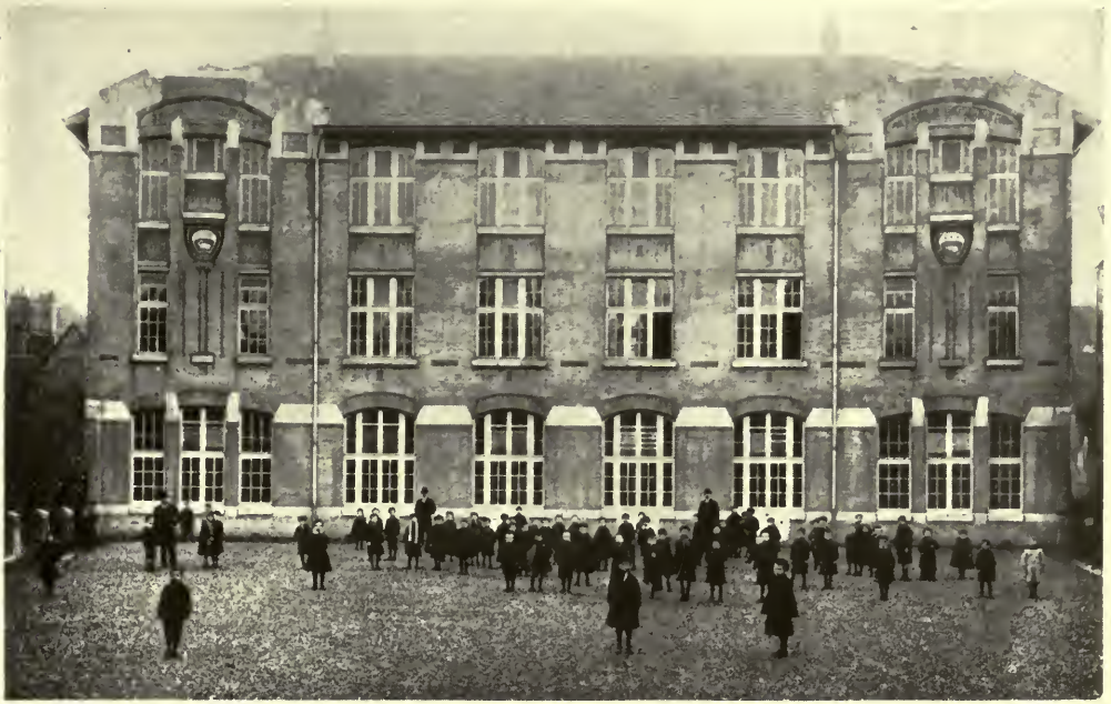
In l'École Communale des Garçons, rue Jean Macé, Le Havre, the open space consists of little more than a walled-in courtyard between the class-room and administration buildings—(see following page)—which is intensively used, however, as an out-of-door class-room and for the gymnastic exercises that are part of the school curriculum. Recreation is a once-a-week affair in the municipal forest on the far outskirts of the city.
