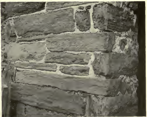
DETAIL OF STONEMWORK OF BARN AT CHEST- NUT HILL, PHILADELPHIA, PA.
