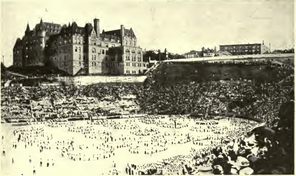
Irregular topography does not necessarily depreciate a school site which rates high in other respects. A gulch between the Tacoma High School Building and Puget Sound provided the opportunity for a stadium with a seating capacity of thirty-two thousand and a field of three and six-tenths acres.
