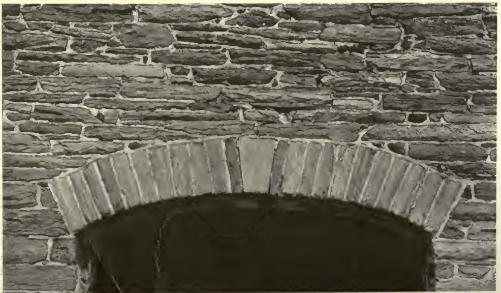
STONEMWORK OF A BARN AT CHESTNUT HILL, PHILADELPHIA, PA.
