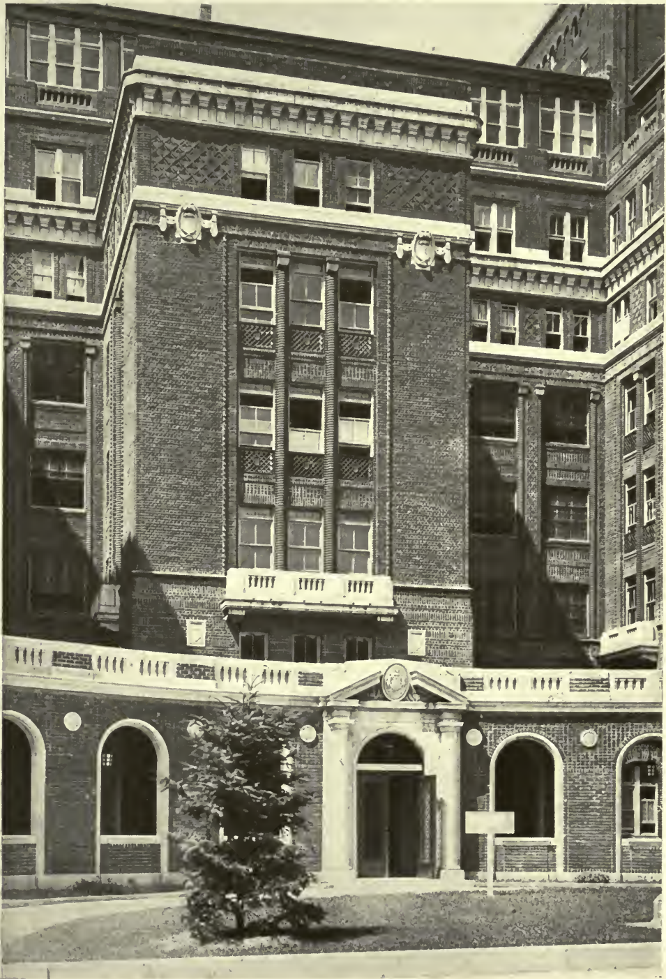
CUMBERLAND STREET HOSPITAL, BROOKLYN. NEW YORK. LUDLOW & PEABODY, ARCHITECTS.
