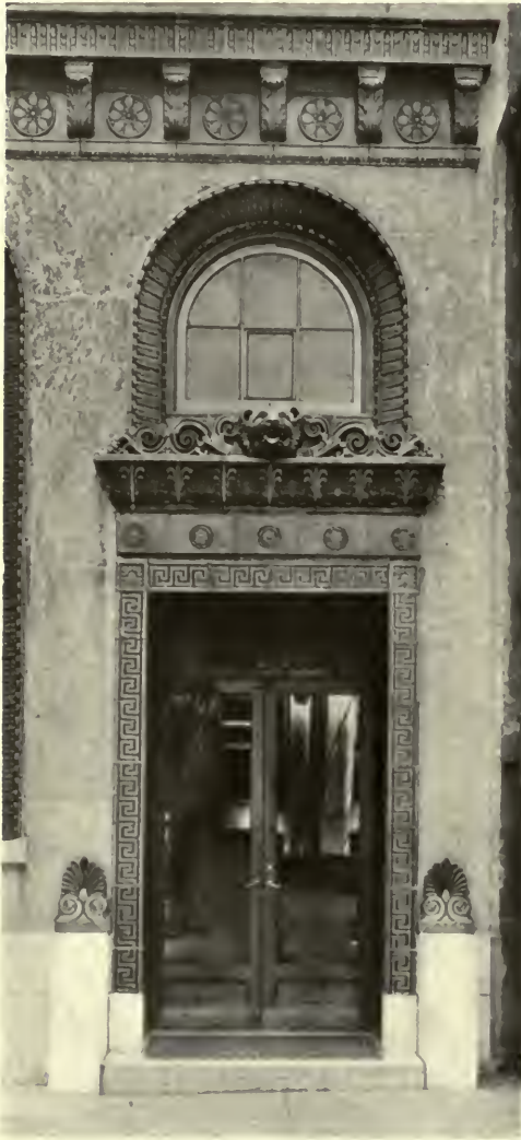
STREET ENTRANCE IN POLYCHROME FAÏENCE, AETCO BUILDING—THE NEW YORK OFFICES OF THE AMERICAN ENCAUSTIC TILING CO.
