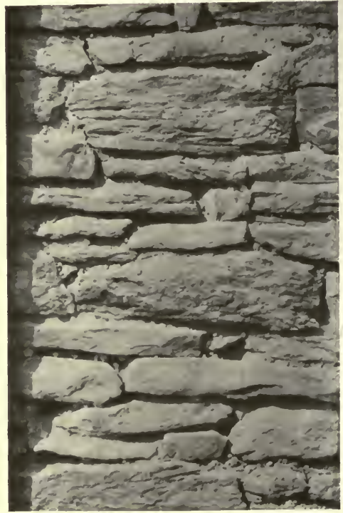
STONEMWORK DETAIL OF ROXBOROUGH HOUSE, PHILADELPHIA, PA.
