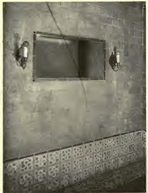
BATHROOM. BASE OF PERSIAN TILE, WALLS OF UNGLAZED BISCUIT TILE. AETCO BUILDING—THE NEW YORK OFFICES OF THE AMERICAN ENCAUSTIC TILING CO.
