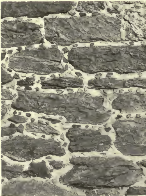
DETAIL OF STONEMWORK WITH "GARRETED" JOINTS, ST. JAMES CHURCH, PHILADELPHIA,
