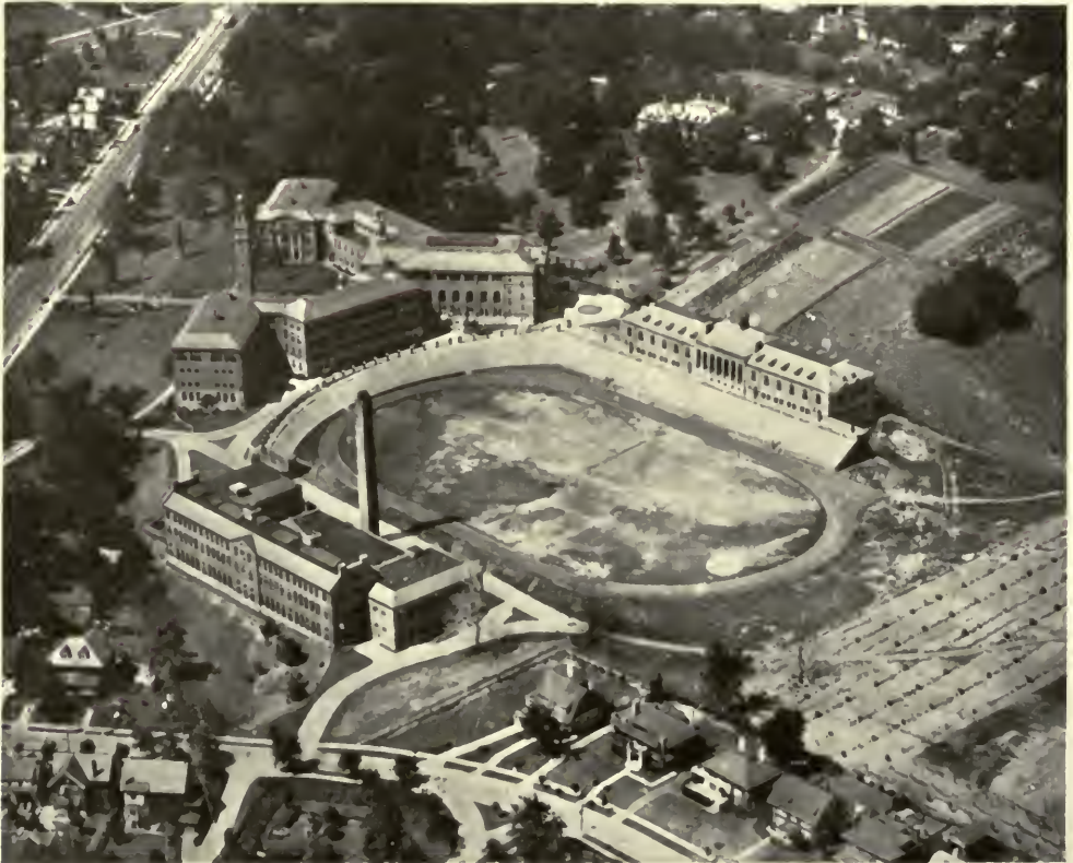
The site of the East Side High School, Cincinnati, Ohio, has sufficient acreage not only for a commodious stadium and athletic field but for a school farm for agricultural instruction.
