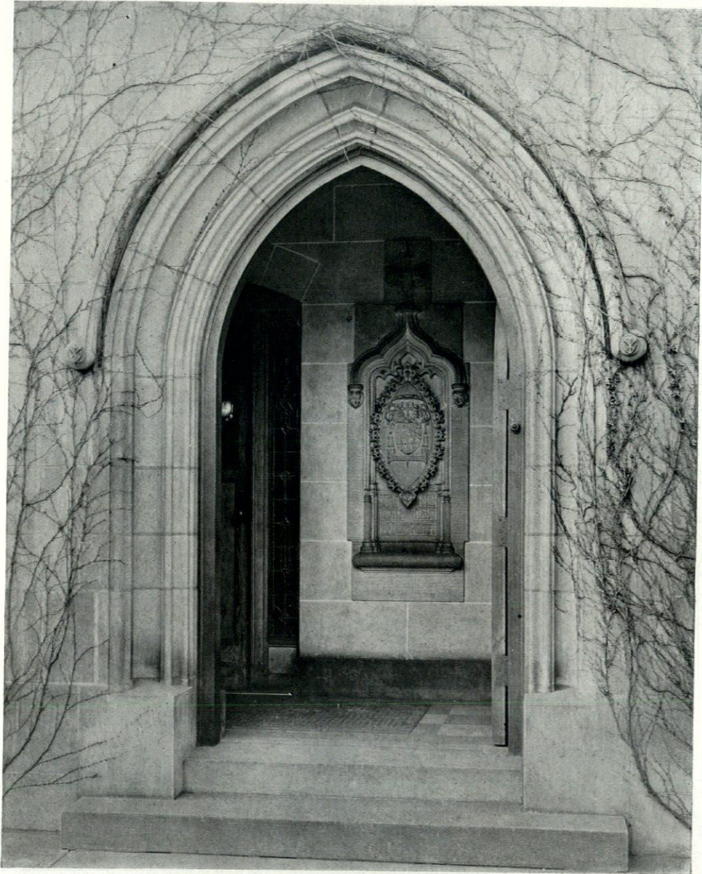
ENTRANCE TO SYNOD HALL AND CHANCERY BUILDING, ST. PAUL'S R. C. CATHEDRAL, PITTSBURGH, PA. — Edward J. Weber, Architect
