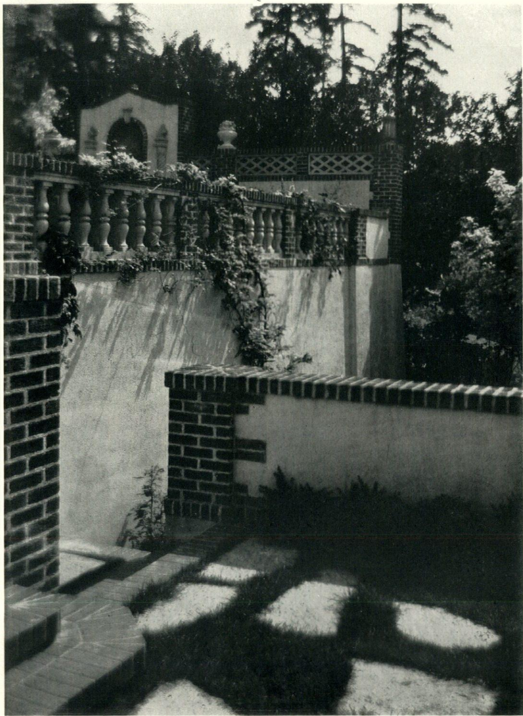
RESIDENCE OF JAMES D. HOGE, ESQ., THE HIGHLANDS, WASHINGTON Bebb & Gould, Architects
