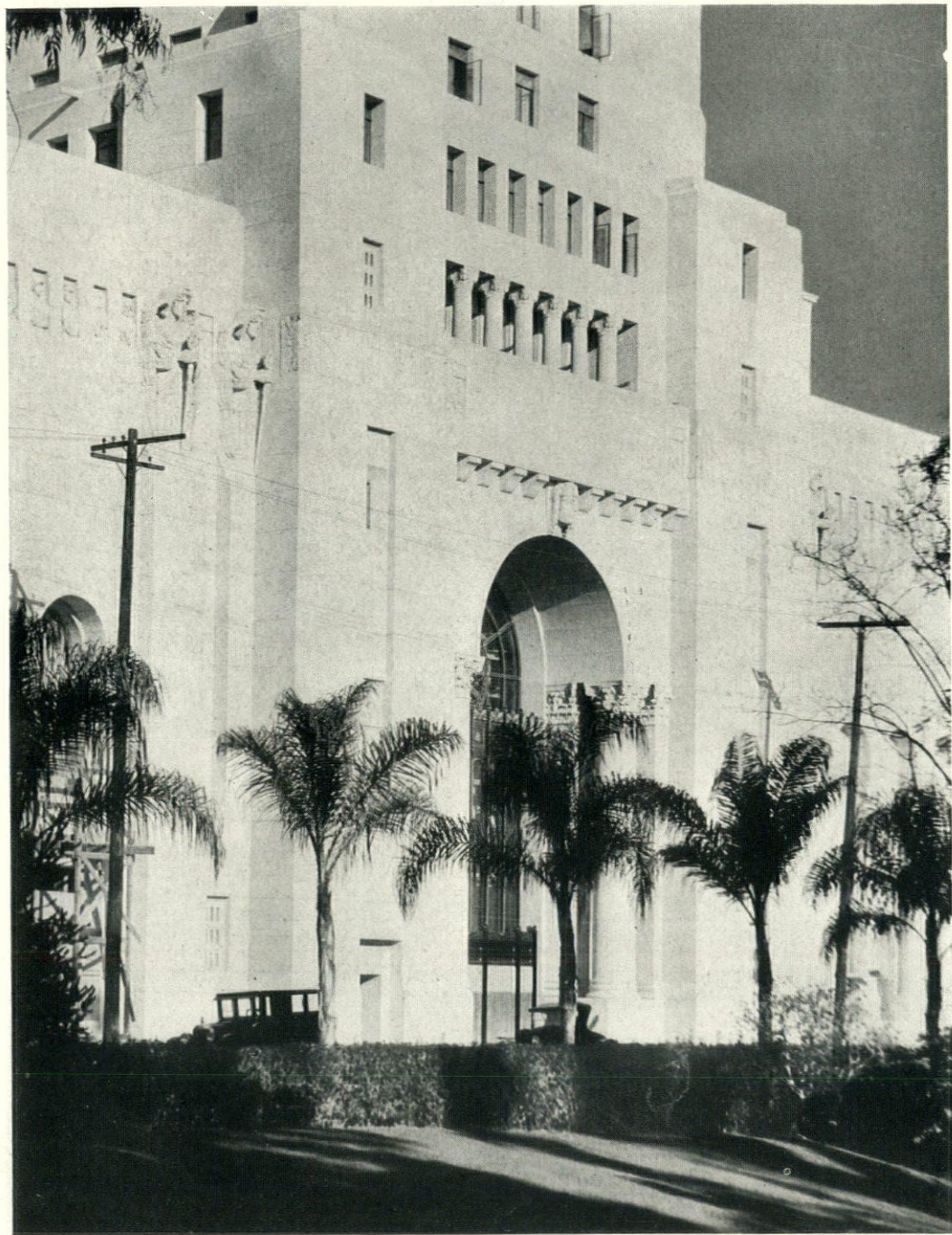
THE ELKS BUILDING, LOS ANGELES, CALIFORNIA Curlett & Beelman, Architects
