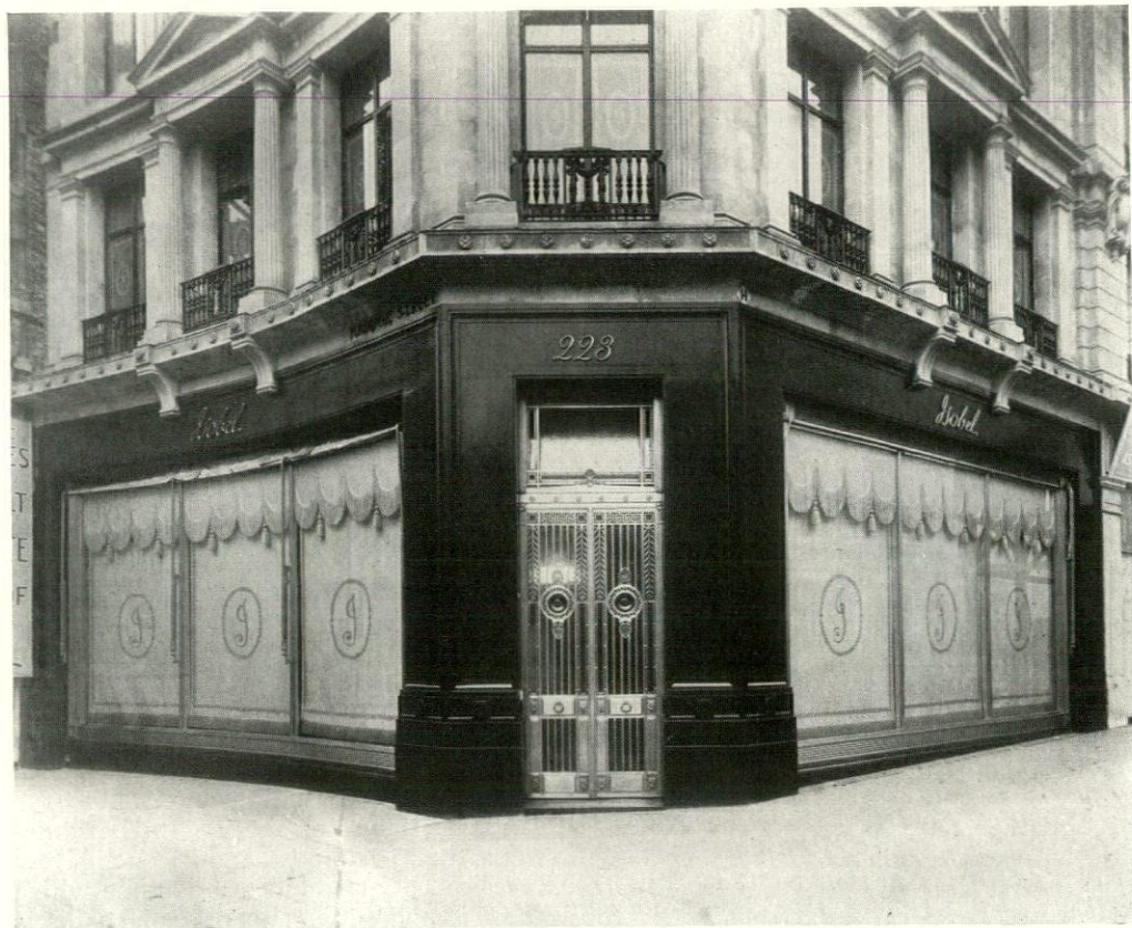
SHOPFRONT OF MADAME ISOBEL IN REGENT STREET, LONDON Carried out in black granite with white metal sashes
