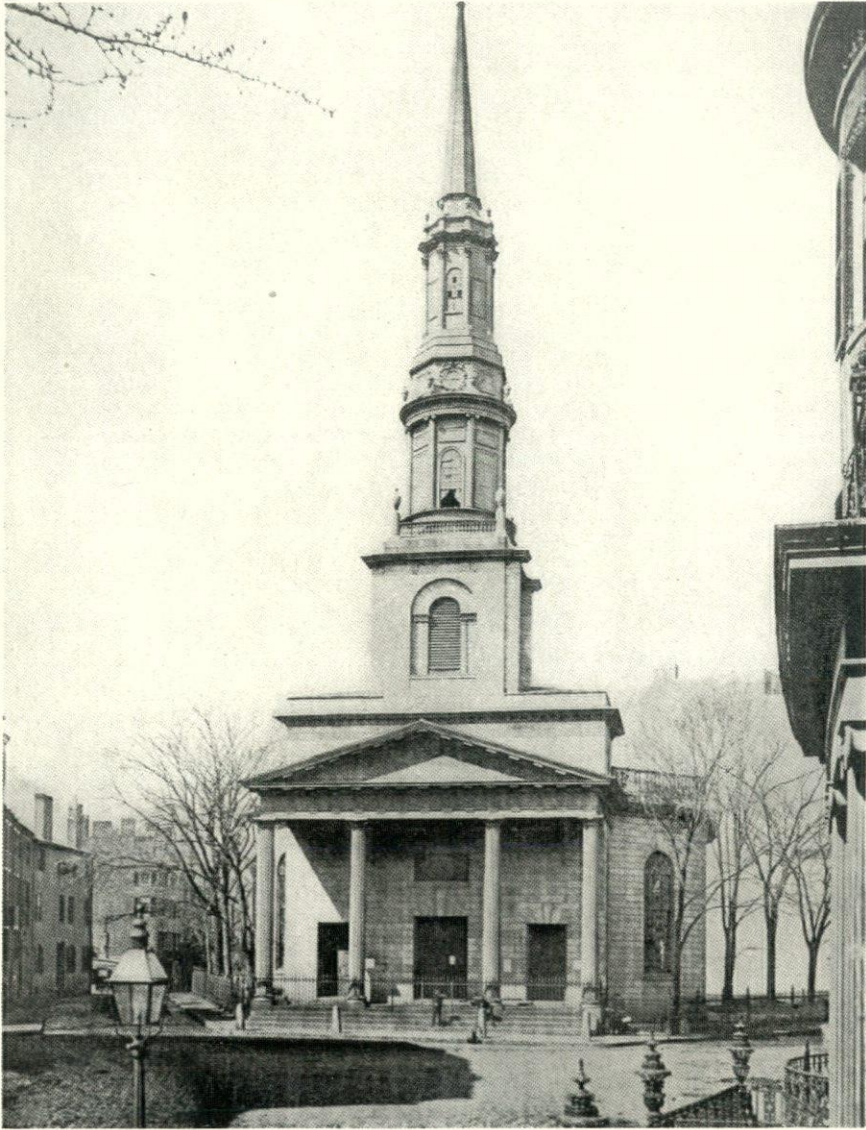
NEW SOUTH CHURCH, BOSTON From Charles Bulfinch, Architect and Citizen .
