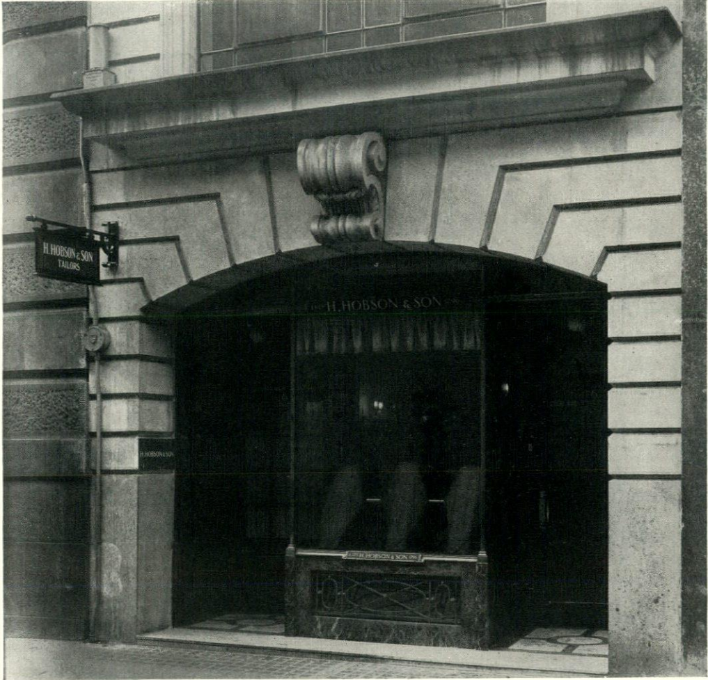
AN EXAMPLE OF A MODERN DOUBLE ENTRANCE FRONT, GRACECHURCH STREET, LONDON
