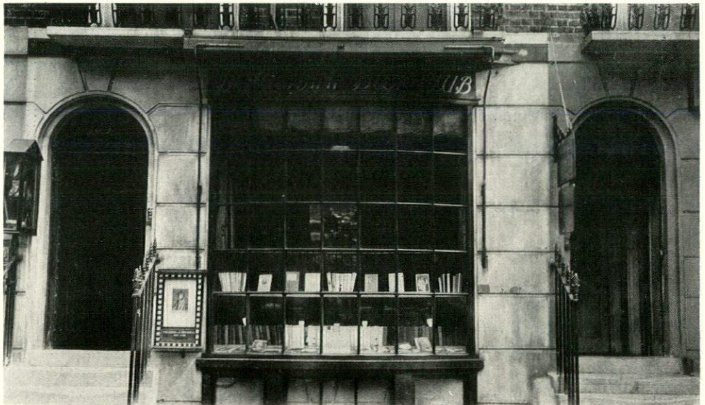
A shop front carried out in mahogany with tiled riser; bevelled glass fanlight over each door with gilt bronze metal grilles
