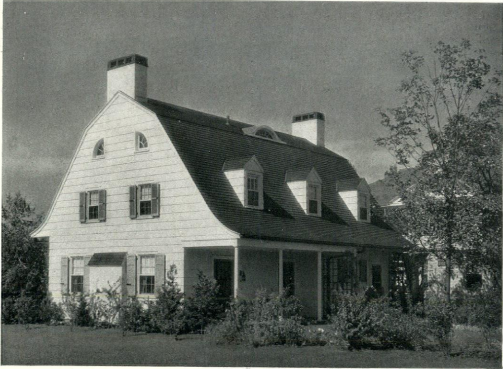
HOUSE FOR W. S. STAIR, ESQ., BELLEROSE, L. I. Lewis E. Welsh, Architect
