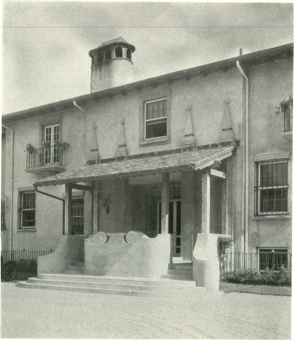
Main Entrance THE DEEPPDALE GOLF AND COUNTRY CLUB, GREAT NECK, LONG ISLAND Warren & Wetmore, Architects
