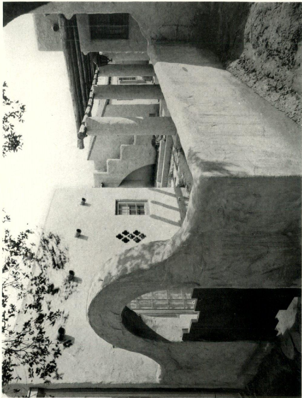
Detail, Patio of the President's House THE KROTONA INSTITUTE OF THEOSOPHY, OJAI VALLEY, CALIFORNIA Robert B. Stacy-Judd, Architect
