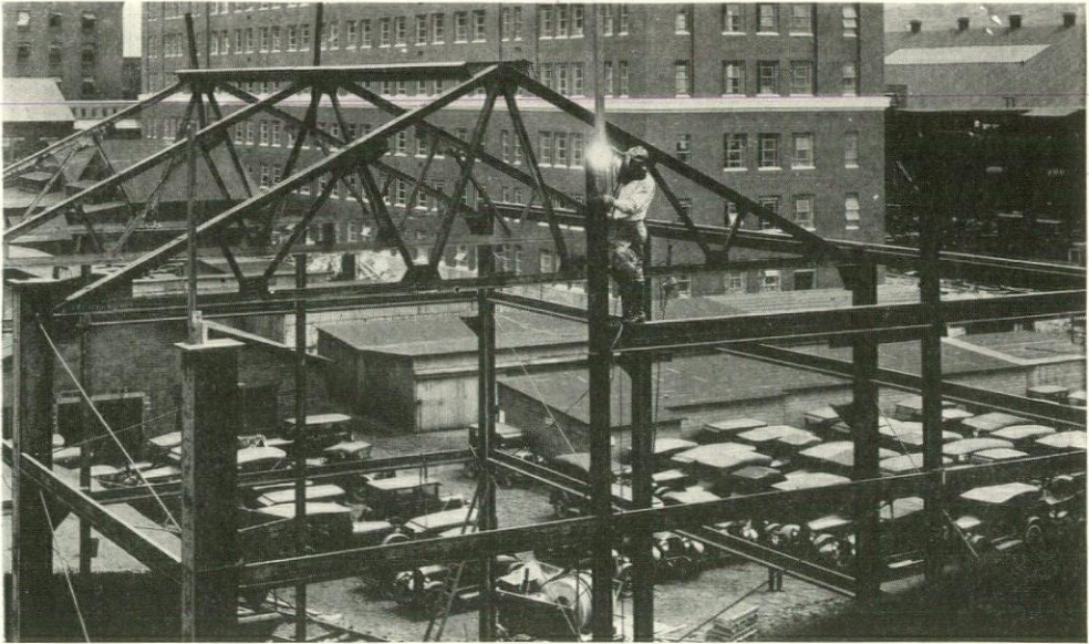
COMPLETELY ARC WELDED BUILDING ERECTED BY THE WESTINGHOUSE ELECTRIC AND MANUFACTURING COMPANY
