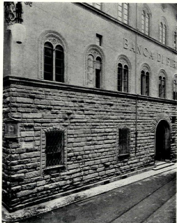
FIG. 84. FAÇADE, PALACE PAZZI-QUARATESI, FLORENCE BRUNELLESCHI, ARCHITECT, 1445
