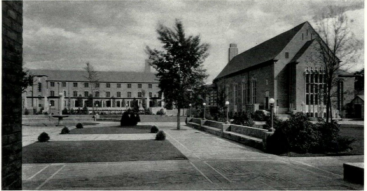
GENERAL VIEW LOOKING FROM ACADEMIC BUILDING
