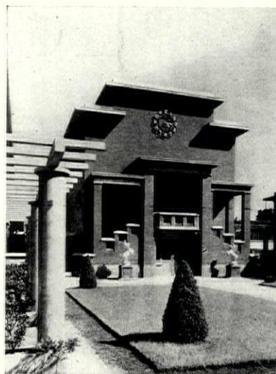
GYMNASIUM AT SURESNES PAYRET-DORTAIL, ARCHITECT From L'Architecture , July, 1928
